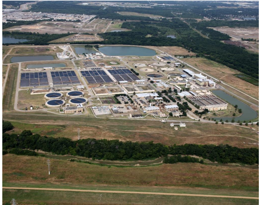
TRA Central Region Wastewater Plant
