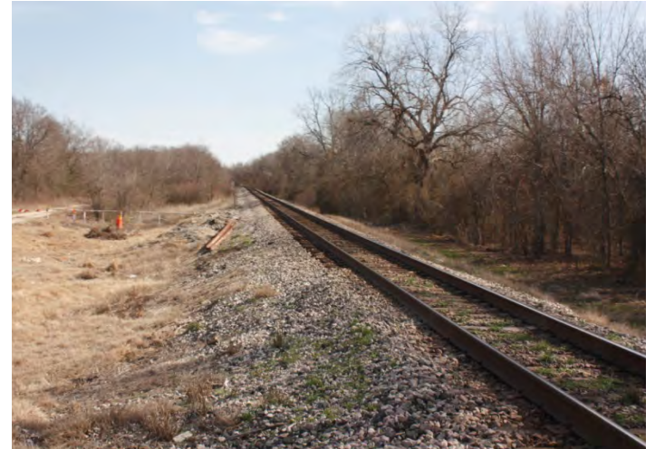
Existing Union Pacific right-of-way at F.M. 875.
