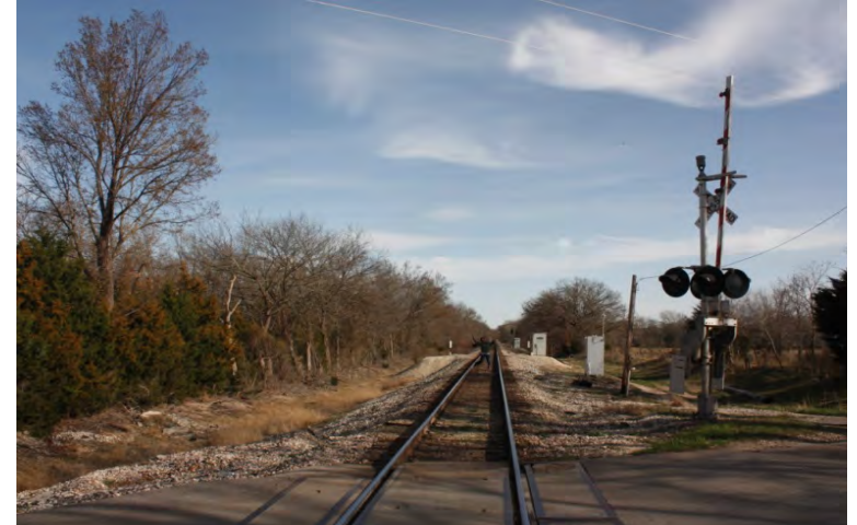
Existing Union Pacific right-of-way crossing Zion Road in Midlothian.
