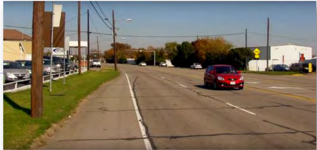
SH 5 Existing Conditions
