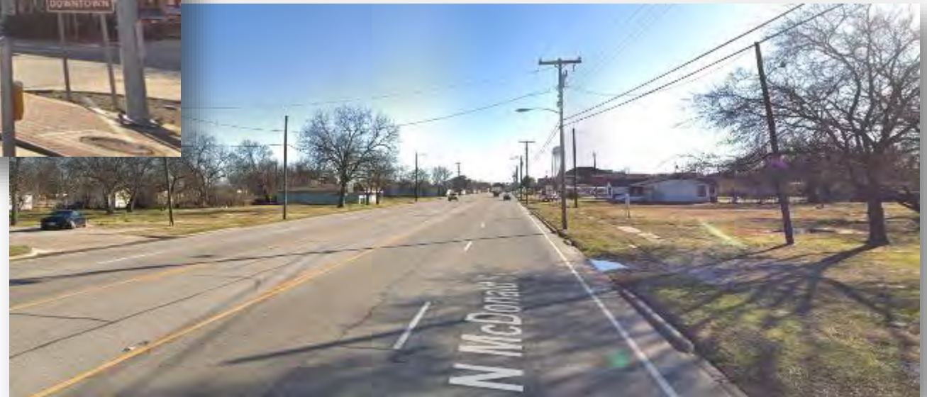
Viewing south on SH 5 @ Watt St
