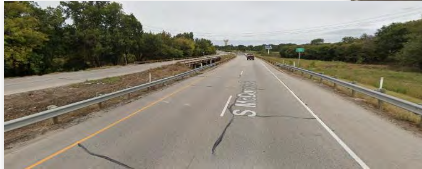
Viewing north on SH 5 @ Wilson Creek
