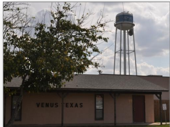
City of Venus Offices and Water Tower
