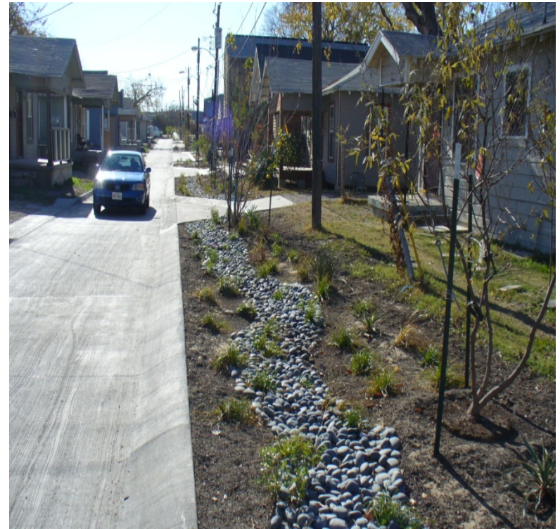
Bioswale and landscaping
