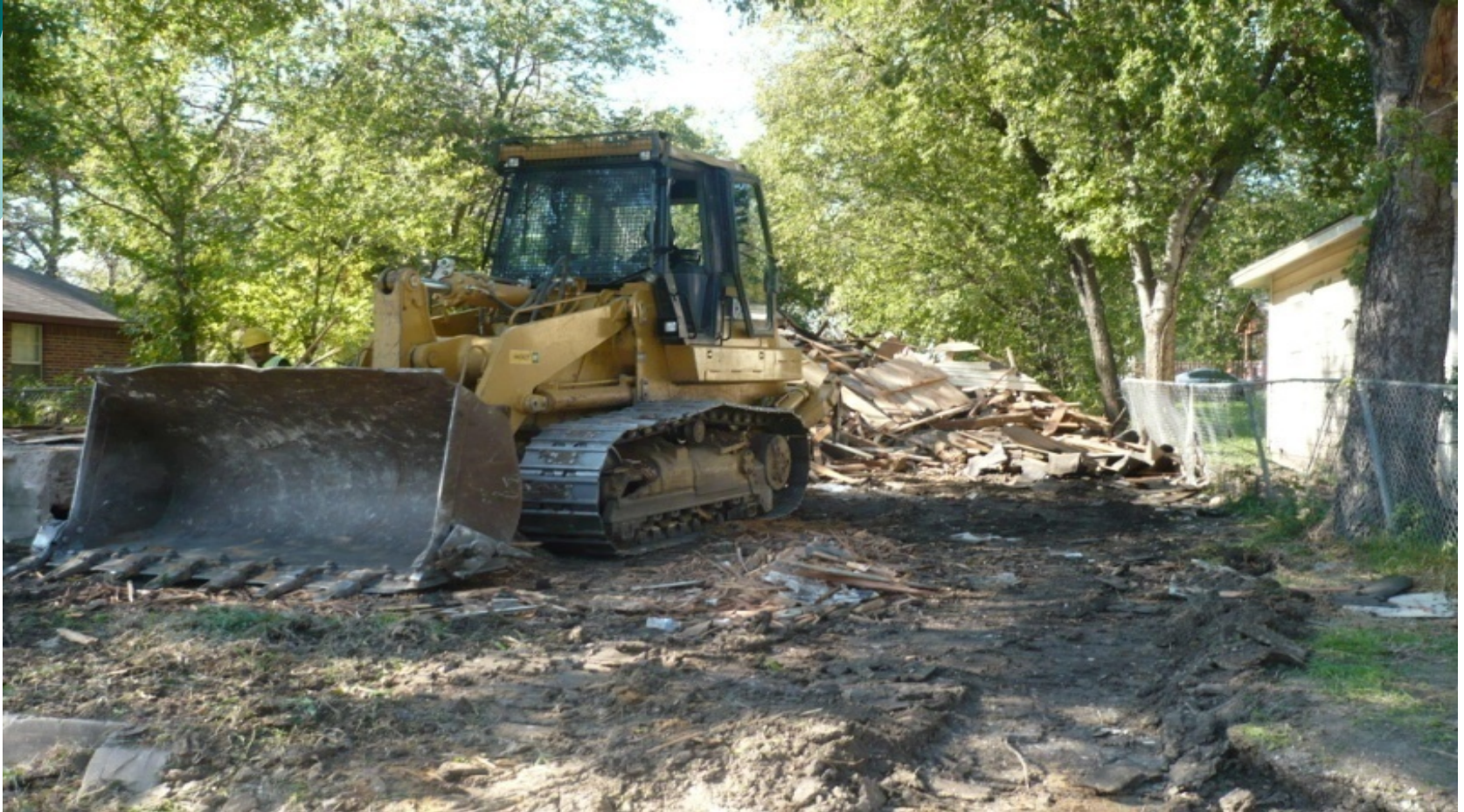
After asbestos abatement-Demolition at 4225 Aztec
