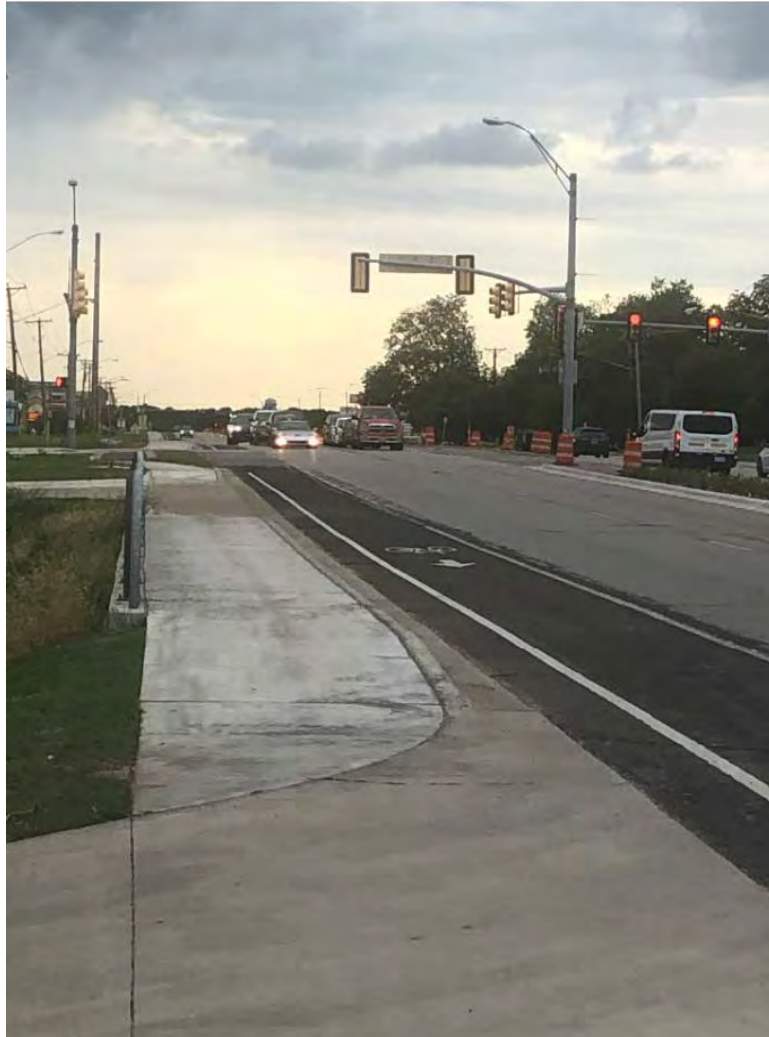
Baker Blvd. Bike Lanes Source: TxDOT Fort Worth District
