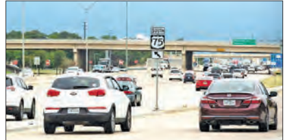
Several developments are under construction along US 75. COURTESY OF THE CITY OF ALLEN
