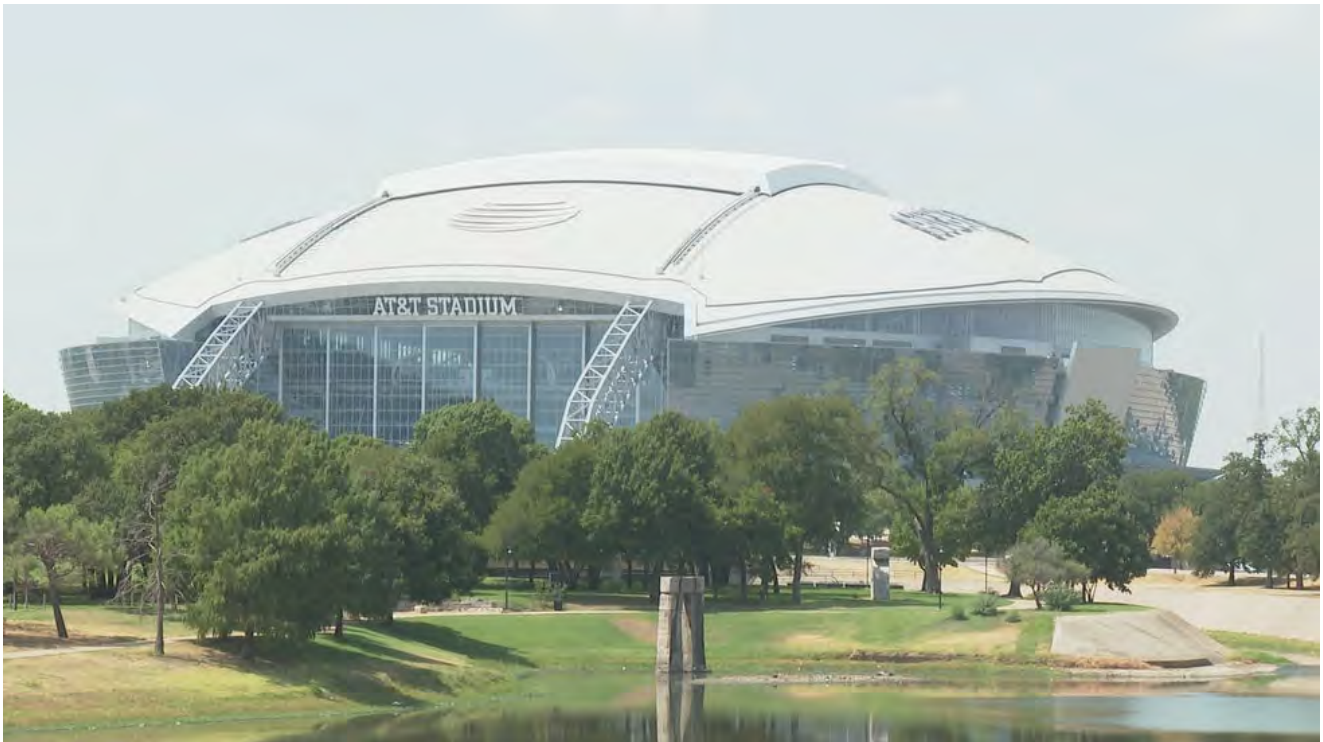
AT&T Stadium, Arlington, TX (KBTX)
