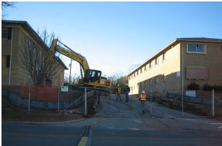
Workers initiate the apartment complex's demolition
