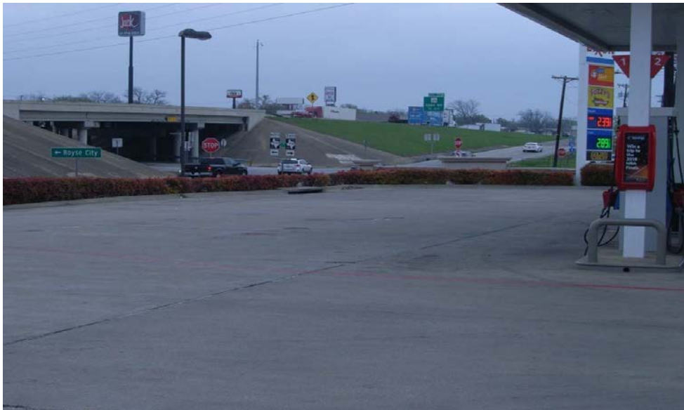
Photograph 48 – View looking northeast near approximate I-30 Sta. 673+50 to 675+50 towards the tank hold of the Tiger Mart 42 gas station LPST and PST site at 117 W. I-30, Royse City, TX (Map ID 18). ROW would be required from the site. The site is considered a moderate environmental risk to the project.
