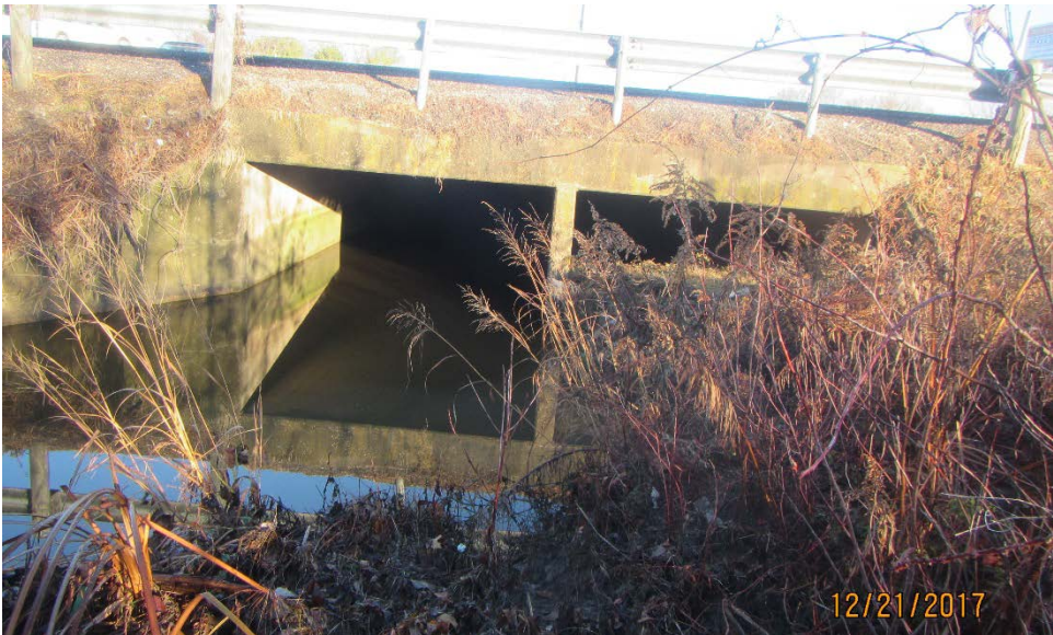
Photograph 2 - View of Stream 2 facing north (eastbound).
