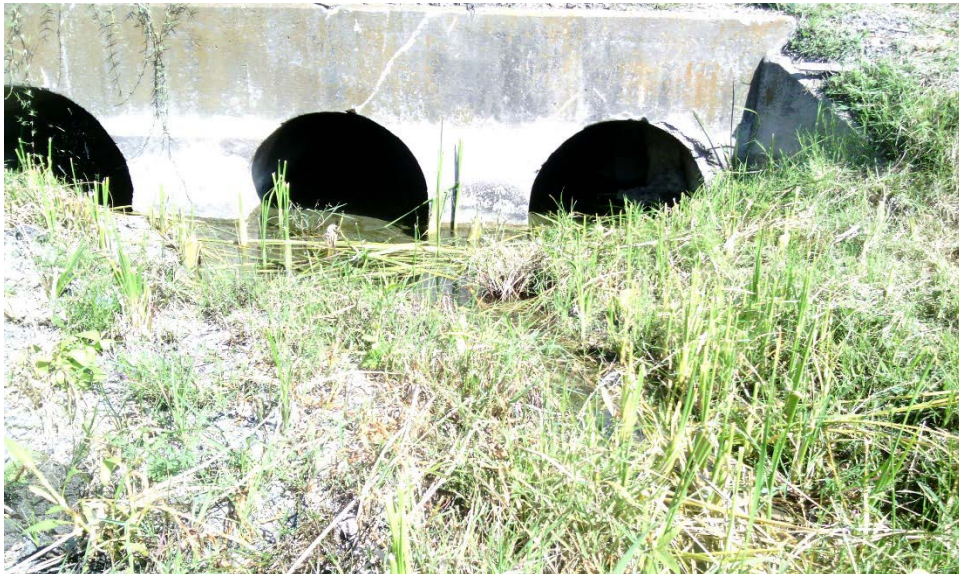
Photograph 10 - View of Stream 6 face northwest (eastbound).
