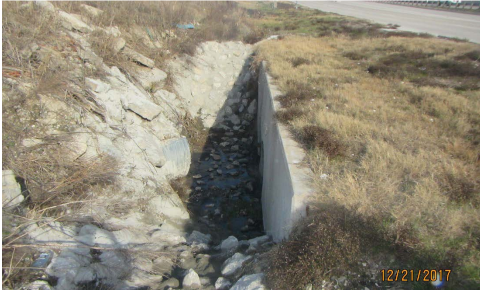
Photograph 11 - View of culvert to Stream 7 facing northeast (westbound).
