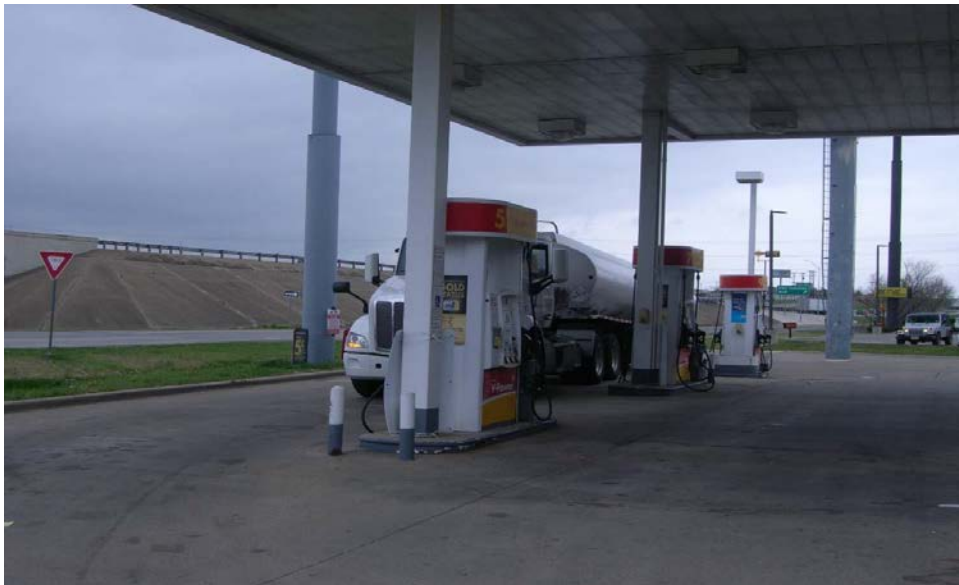
Photograph 50 – View looking southwest near approximate I-30 Sta. 676+50 to 678+00 towards the pump island and tank hold of the Triple C Convenience Store and gas station LPST and PST site at 100 W. I-30, Royse City, TX (Map ID 24). No ROW would be acquired from the site. The site is considered a high environmental risk to the project.
