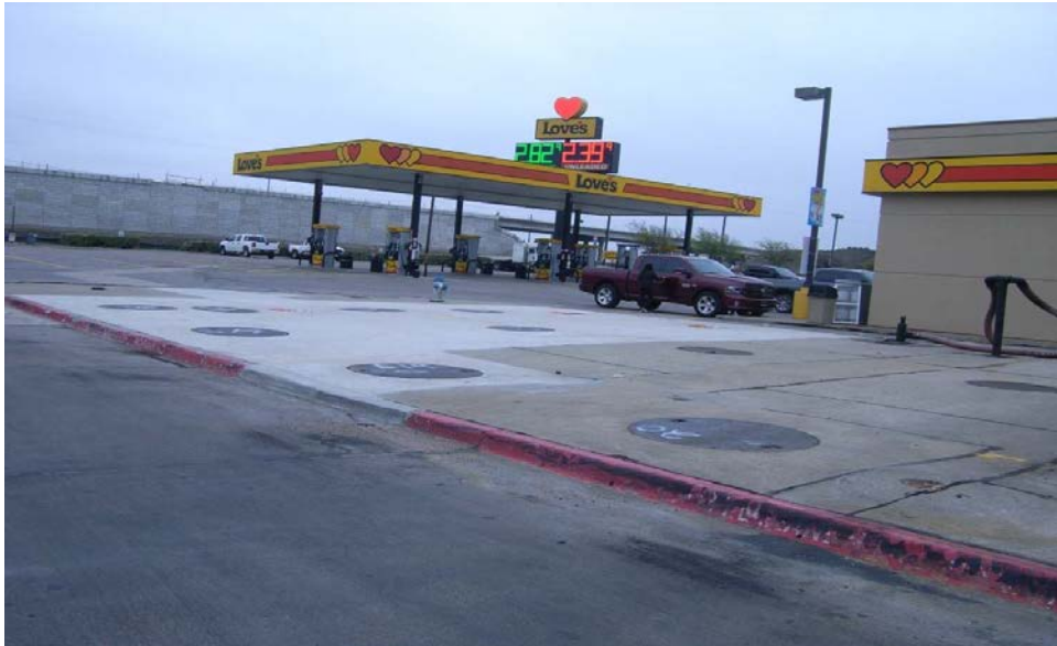
Photograph 51 – View looking northeast towards one of two tank holds of Loves Country Store 283 gas station LPST and PST site at 1990 E. I-30, Rockwall, TX (Map ID 45). I-30 is in the background of the photo and the pump islands in the photo serve automobiles and small trucks. ROW would be acquired from the site. The site is considered a moderate environmental risk to project
