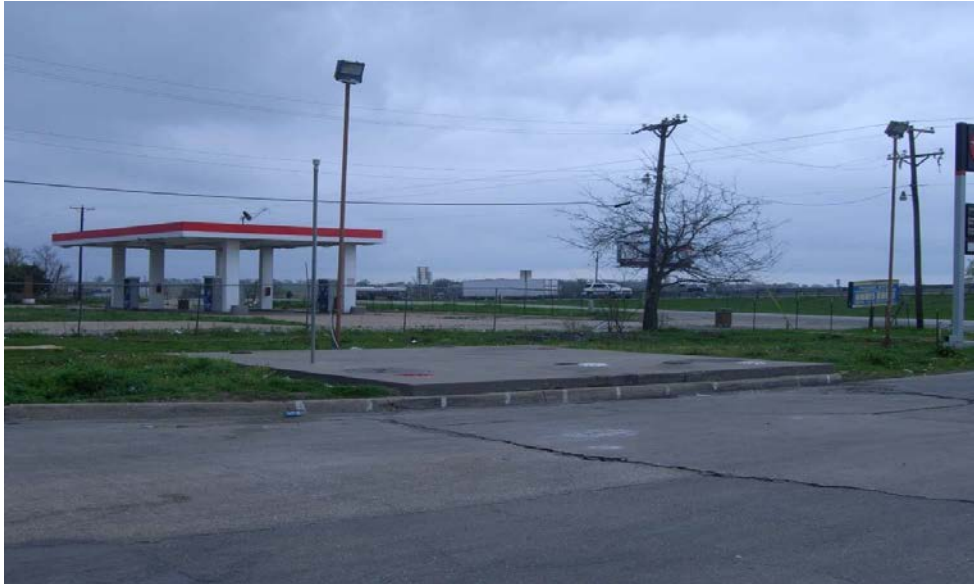
Photograph 47 – View looking east-southeast near approximate I-30 Sta. 714+00 towards one of two tank holds of the Sunmart 106 PST site at 926 E. I-30, Royse City, TX (Map ID 11). This tank hold serves automobiles and small trucks at pump islands (right of the photo out of view). ROW would be acquired from the site. The former Prime Travel Stop gas station is in the background of the photo. The site is considered a moderate environmental risk to the proposed project.
