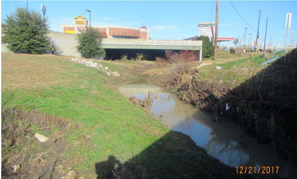
Photograph 21 - View of Stream 13 facing northwest at FM 548.
