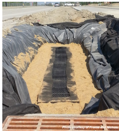
Installation of Bioretention Green Infrastructure on Merritt Road in Rowlett, TX
