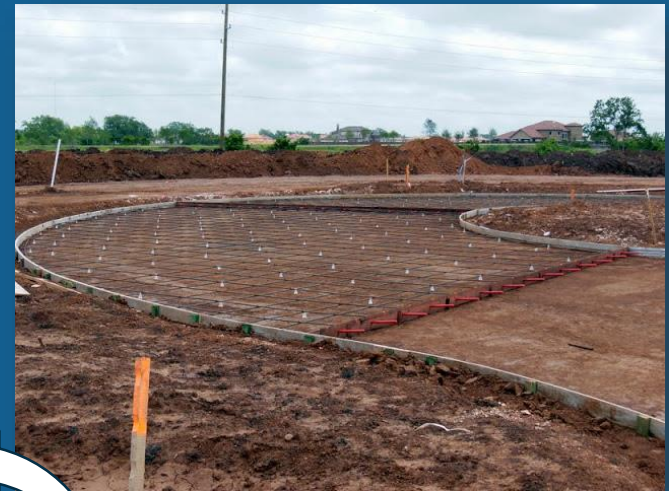
Jointed Reinforced Concrete Pavement (JRCP)
