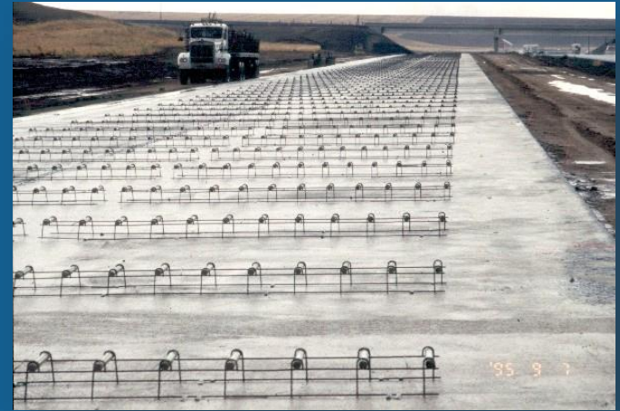
Jointed Plain Concrete Pavement (JPCP)
