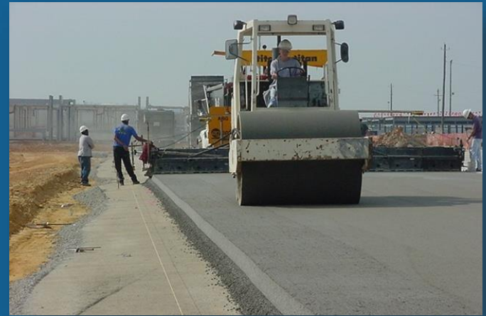
Roller Compacted Concrete Pavement (RCCP)
