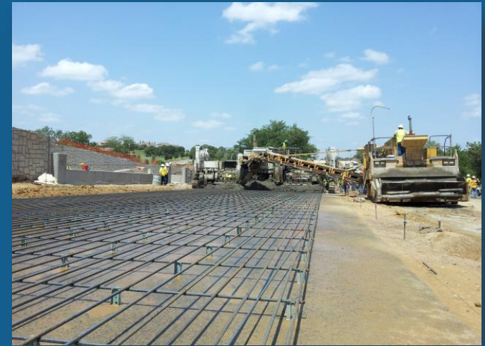
Continuously Reinforced Concrete Pavement (CRCP)
