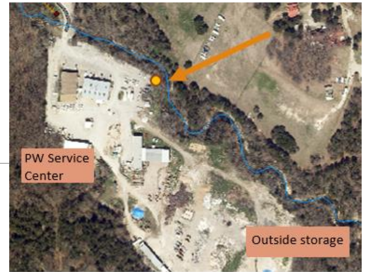
Public Works "Service Center" has open drainage channel that discharges to trib. of Red Oak Creek
