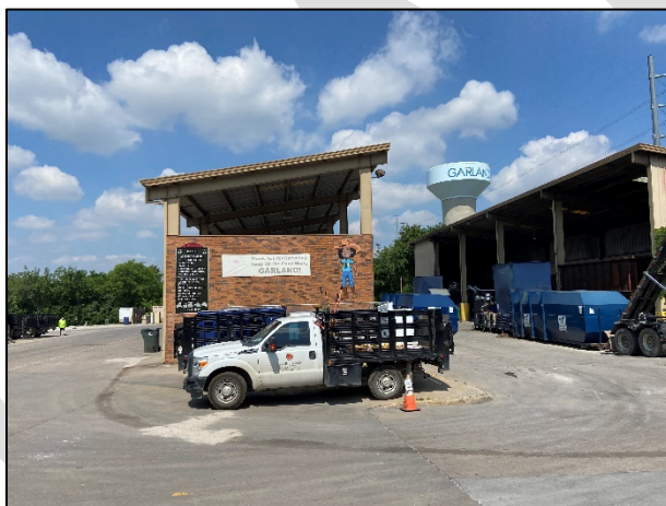
Figure 5-5: Example of Equipment Configuration Blocking Recycling Center Operations
