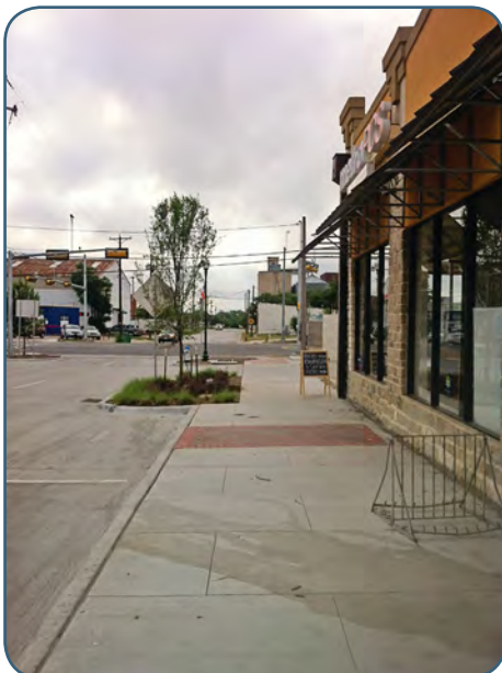
Recent Virginia Street Improvements
