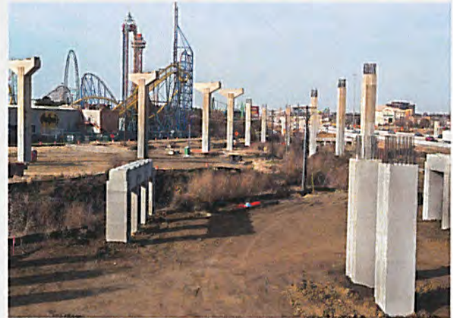
Bridge column construction on the I-30/SH 360 Interchange Project in Arlington. The $233 million project will increase safety, connectivity and mobility for motorists.
