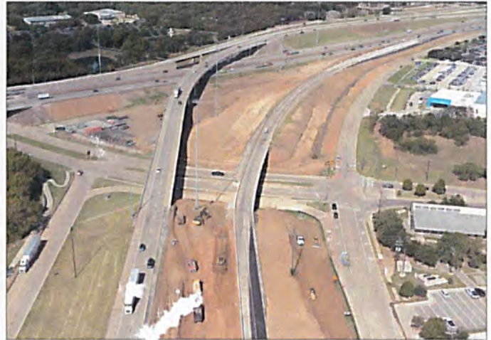
SH 121/360 interchange construction
