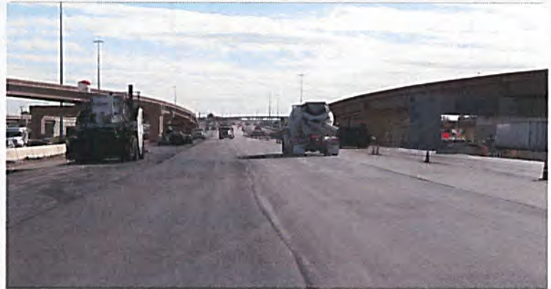
Nov. 2016 - Future I-35W TEXpress Lanes at Western Center Boulevard
