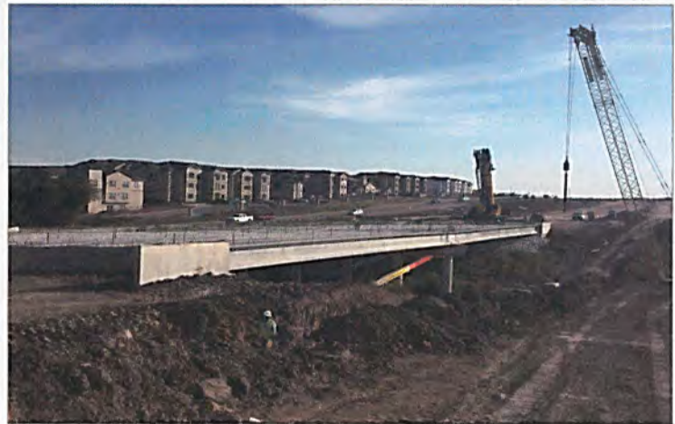
November 2016 - Future SH 360 bridge over Bowman Branch
