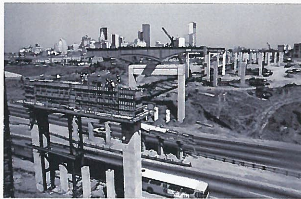
At Left: I-345 under construction in 1969. Credit: The Dallas Library
