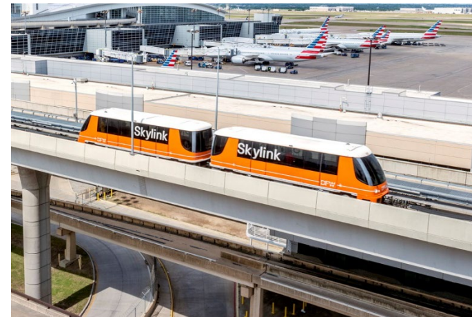
Skylink people mover trainset in operation at Dallas Fort Worth International Airport. (Source: Dallas Fort Worth International Airport, 2014)
