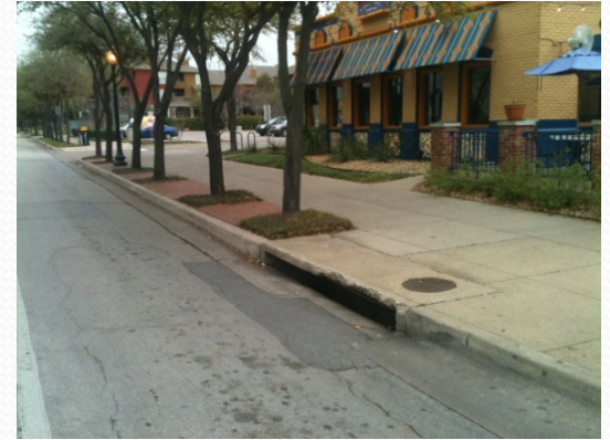
The old way of thinking – deliver water to storm inlet as quickly as possible and do not nourish nearby trees
