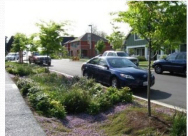
A bioswale and permeable concrete are used for stormwater management and to enhance neighborhood aesthetics (Source: Abby Hall, US EPA)
