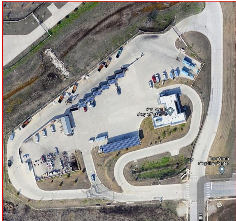
Figure 3-3 In 2020, the City of Fort Worth Hillshire Drop-off Center
