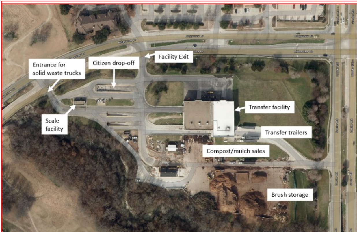
Figure 3-10 NTMWD Custer Road Transfer Station (Plano, Texas)
