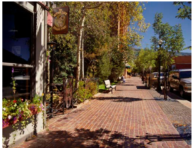
Image 34: Pedestrian spaces should require greater attention to details such as paving, lighting, and furniture choices.
