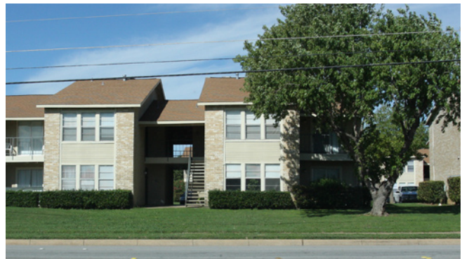
Image 3: Existing two-story apartment buildings are found throughout the Study Area.
