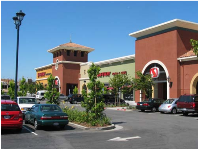
Image 31: Enhanced and landscaped outdoor parking areas provides greater comfort and benefit to pedestrians and the vehicular environment.
