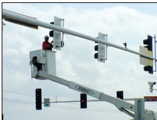
Traffic signal improvements help minimize delays at intersections.
