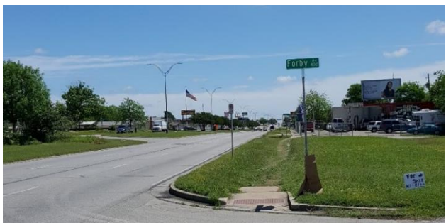
Existing conditions showing unprotected and sporadic sidewalks, wide median, and existing land uses.
