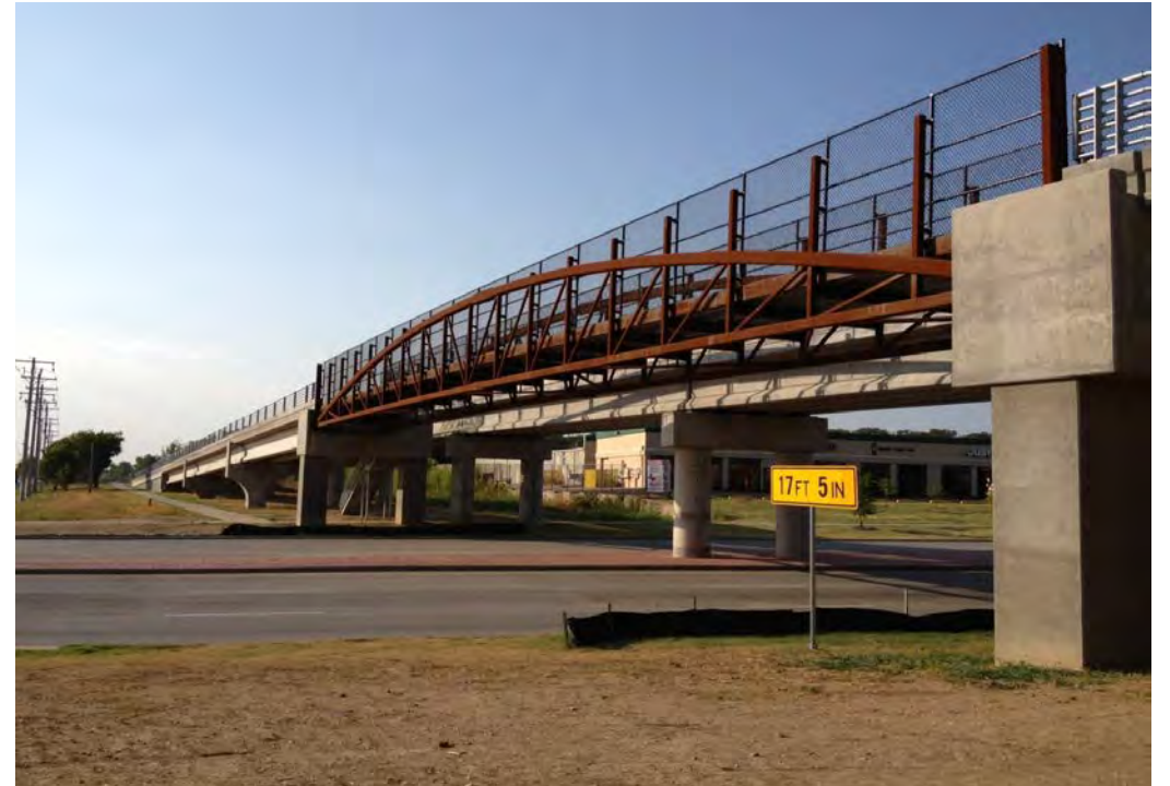
Photo Courtesy City of Denton: MLK Trail Bridge at Loop 288 constructed adjacent to the DCTA Rail Bridge
