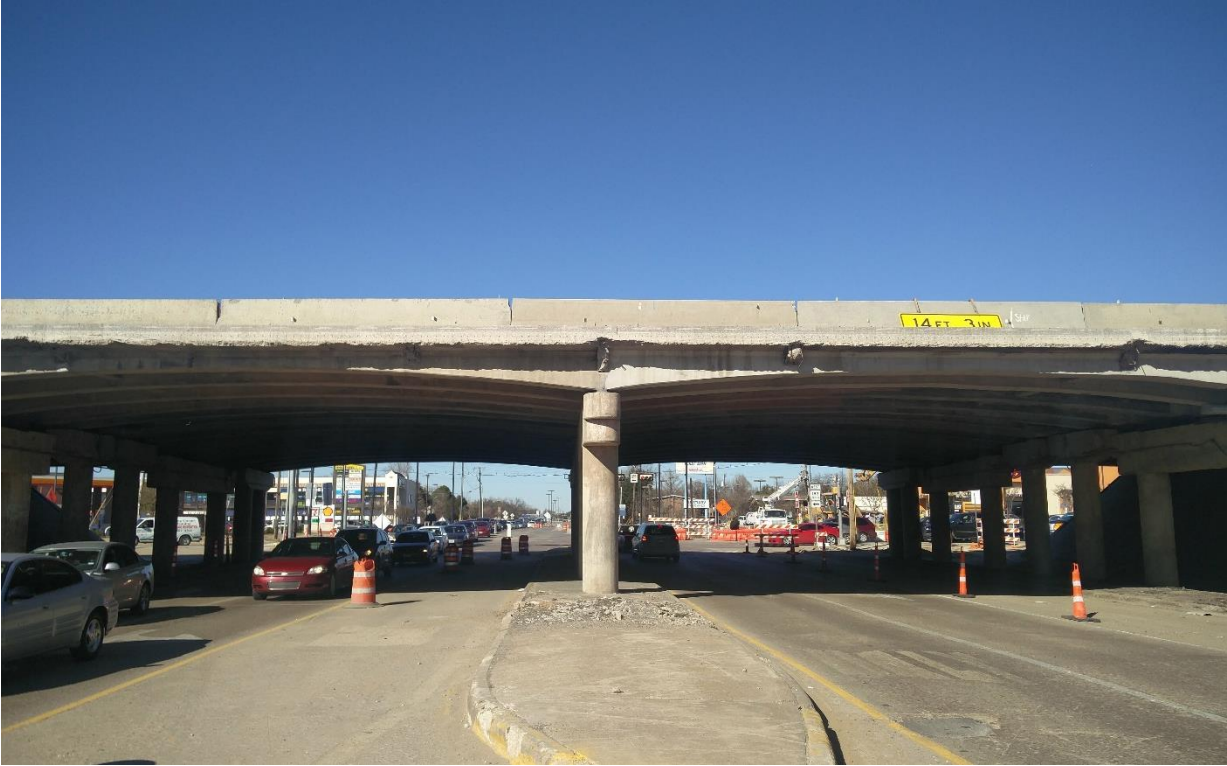
SH183 Over MacArthur Boulevard, Irving
