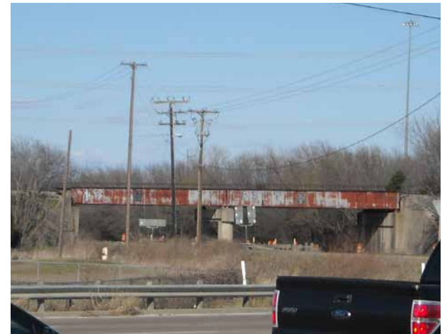
Figure 4.11 (Top) Existing Area 4 Development
