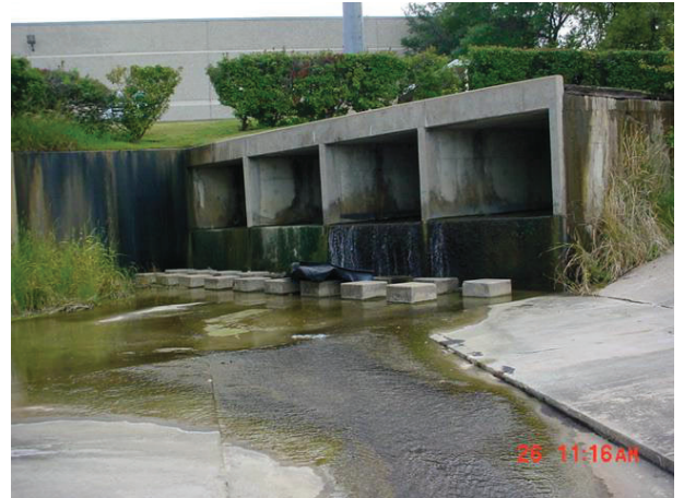
Photo facing upstream - culverts crossing under I-30
