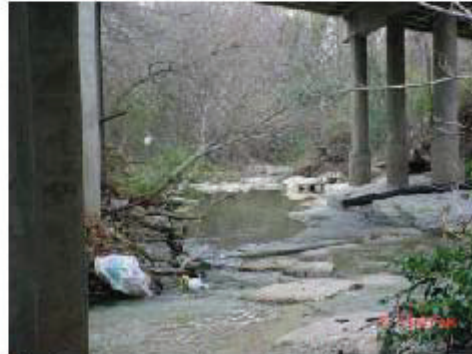
Facing downstream of sample reach
