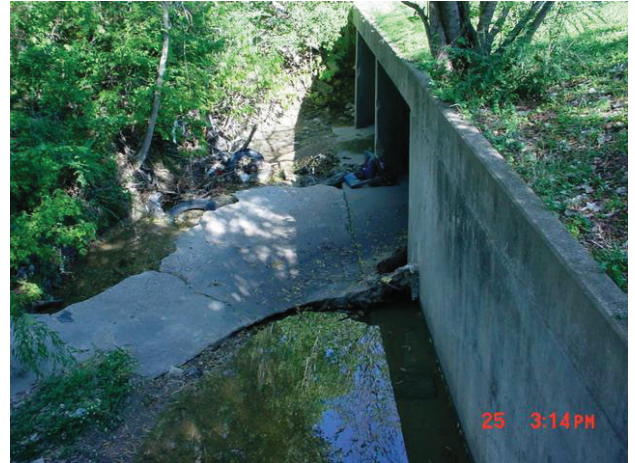
Sample site – downstream side of the Linfield Rd. bridge
