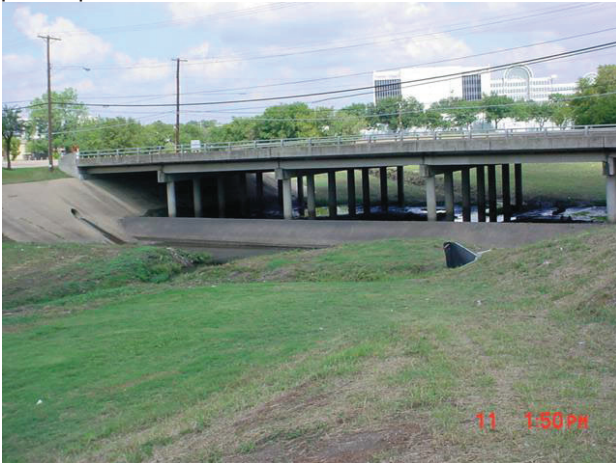
Facing upstream - Market Center Blvd shown in the distance
