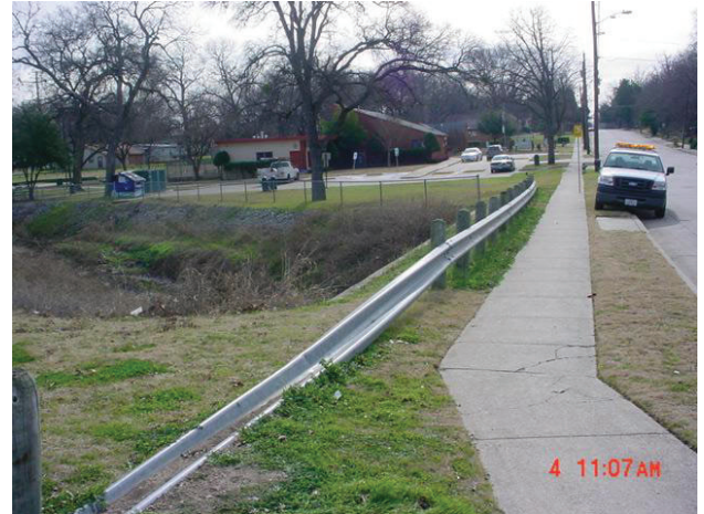
Sample site access point
