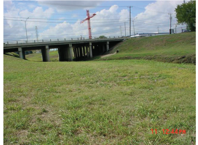
Facing downstream with Irving Blvd. in the distance
