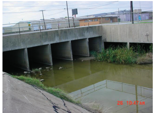
Photo facing upstream from sample area
