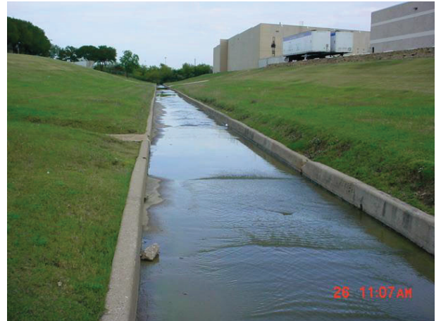
Photo showing downstream side of sample area
