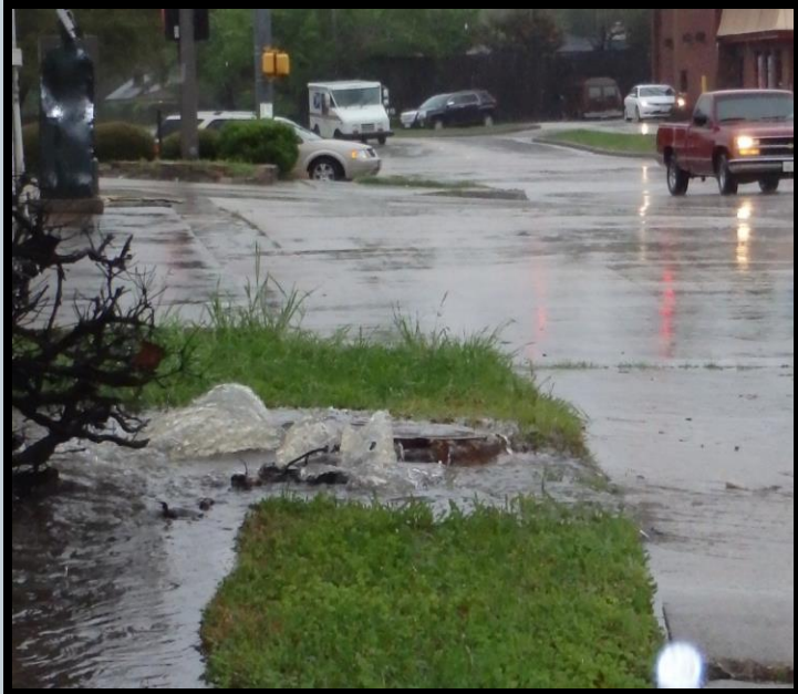
SANITARY SEWER OVERFLOWS
