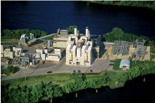
Figure 6 - Fluidized Bed RDF Combustion, Wisconsin
