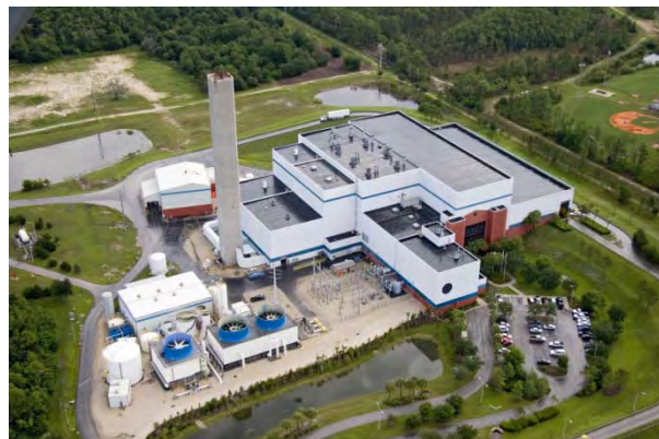
Figure 7 - Mass Burn Facility, Florida
