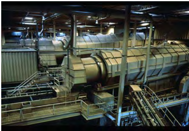
Figure 3 - RDF Processing Facility, Virginia
