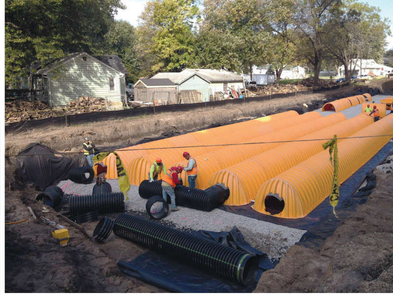
Soakage Trench installation. (Source: Wikipedia, CC BY-SA 3.0)
