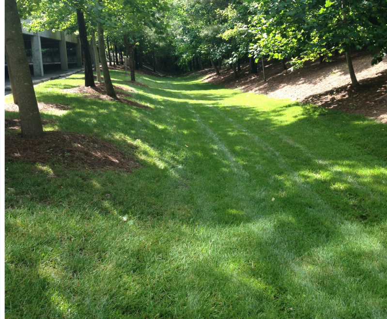
Grass Channel in Durham, NC. (Source: Tetra Tech)
