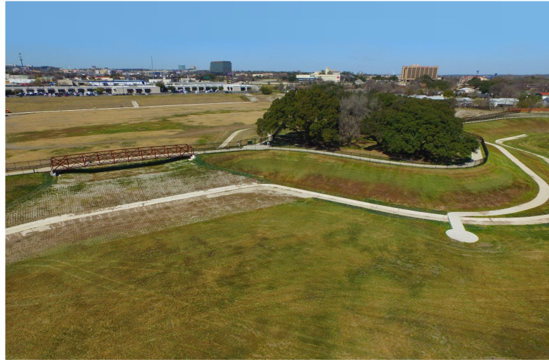
Dry Detention Facility in San Antonio, TX. (Source: Halff)
