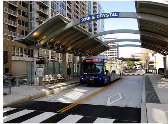
Metroway Station (Source: Arlington, Virginia)
