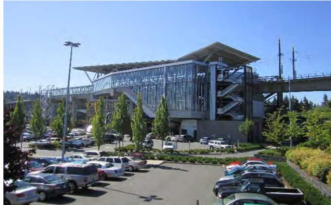
Tukwila International Boulevard Station (Source: Seattle, Washington)
