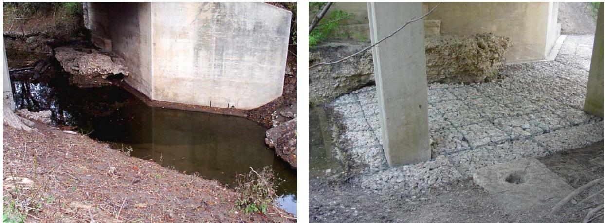
Figure 25. Erosion Repair and Scour Protection (Gabion Mattresses).
