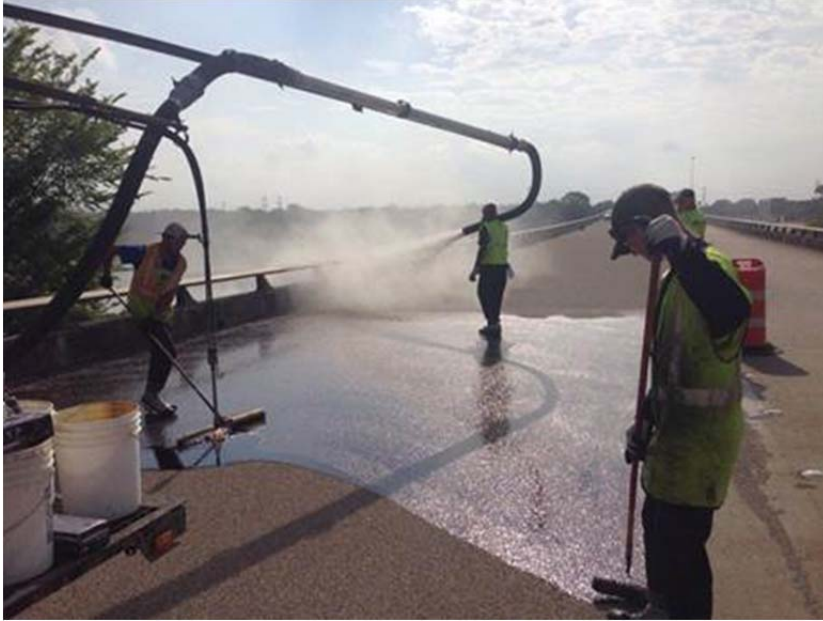
Figure 35. Application of Polymer Overlay Deck Surface Treatment Project (SH 31 WB over Trinity River in the Tyler District).
