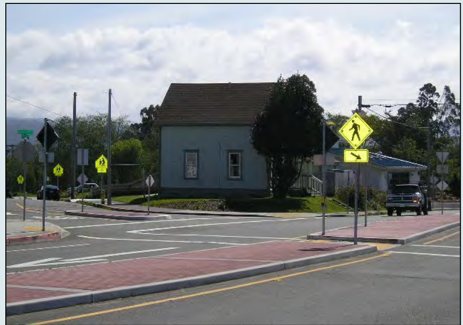
Intersection with the permanent improvements
