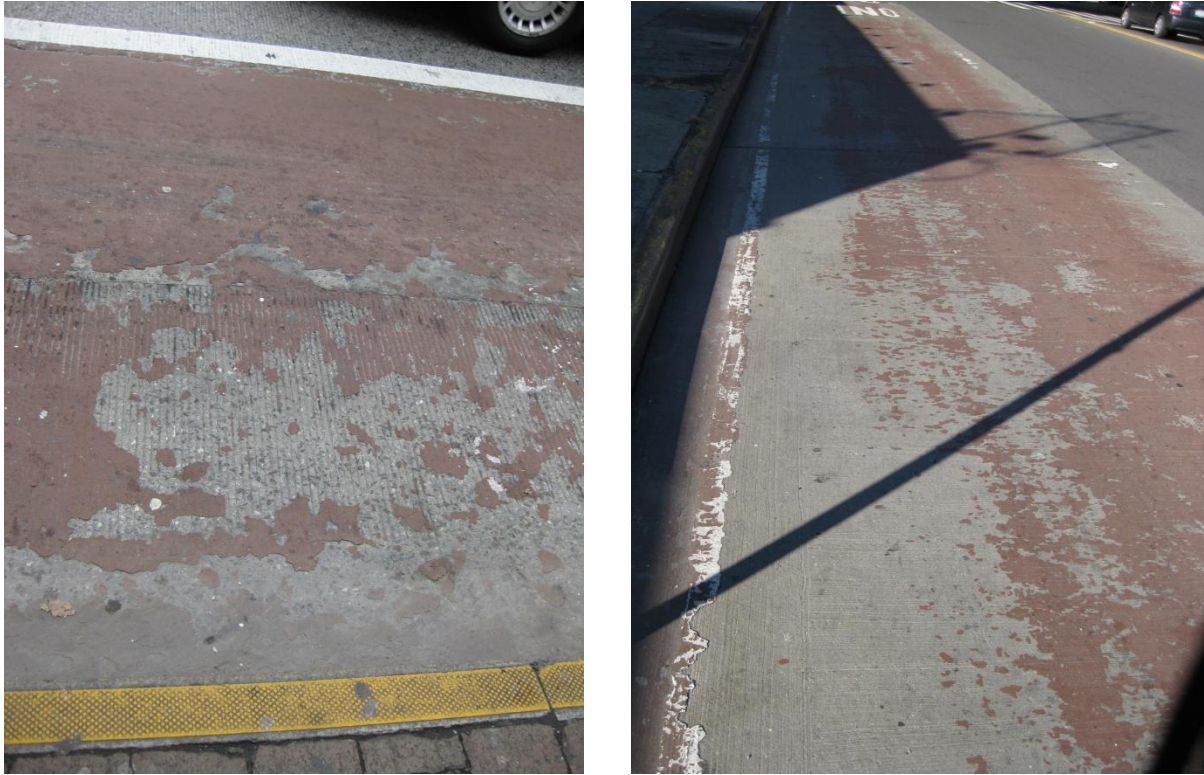
Figure 5. Product ID #1 on concrete roadway in the vicinity of Sedgwick Avenue on Fordham Road after one year (left), red treatment concrete roadway at West 207 th Street at Tenth Avenue after one year (right)
