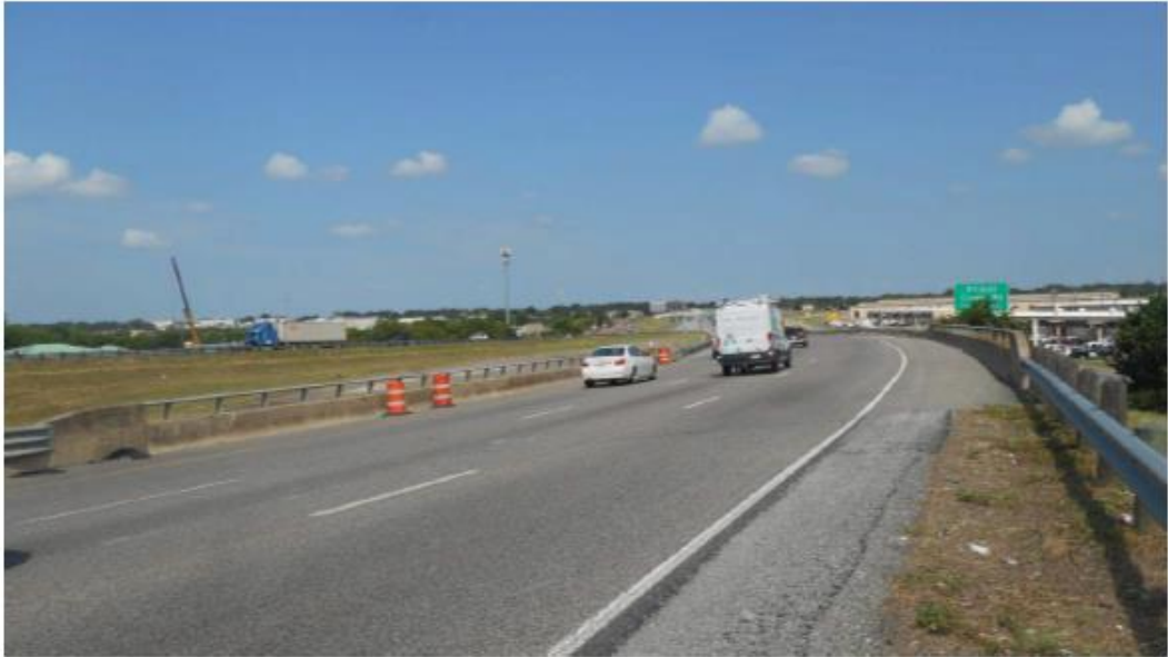
1 - Roadway looking North
