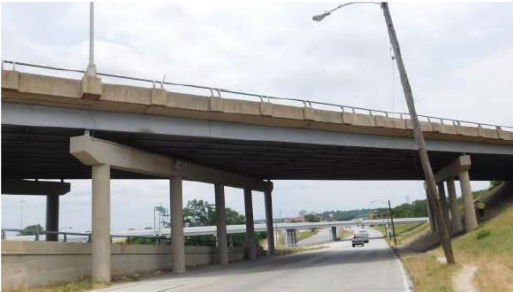
4 - Roadway Under looking East (Lancaster EB)
