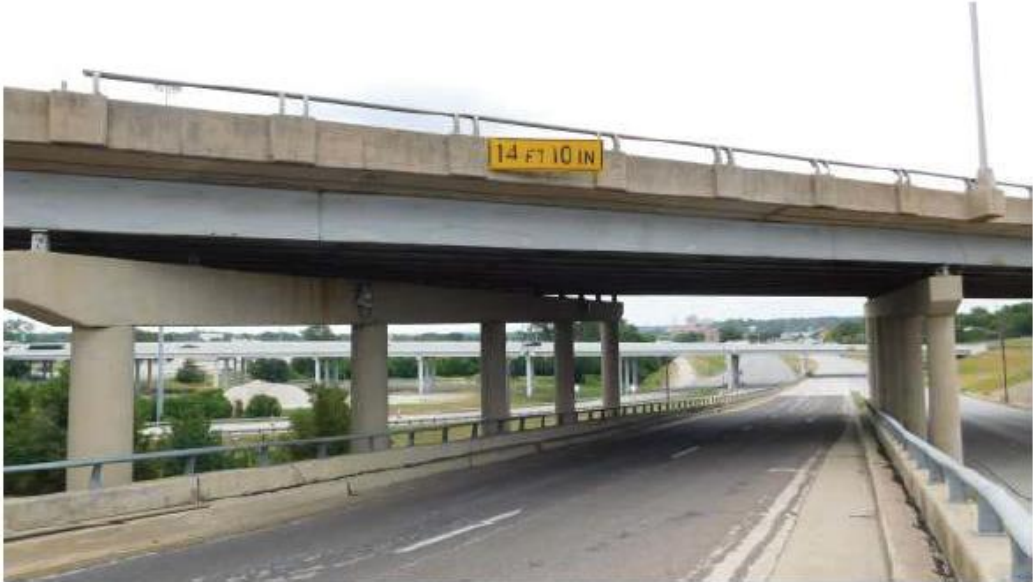
5 - Roadway Under looking East (Lancaster EB Ramp)
