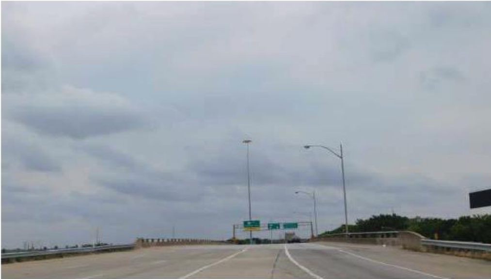
1 - Roadway looking South
