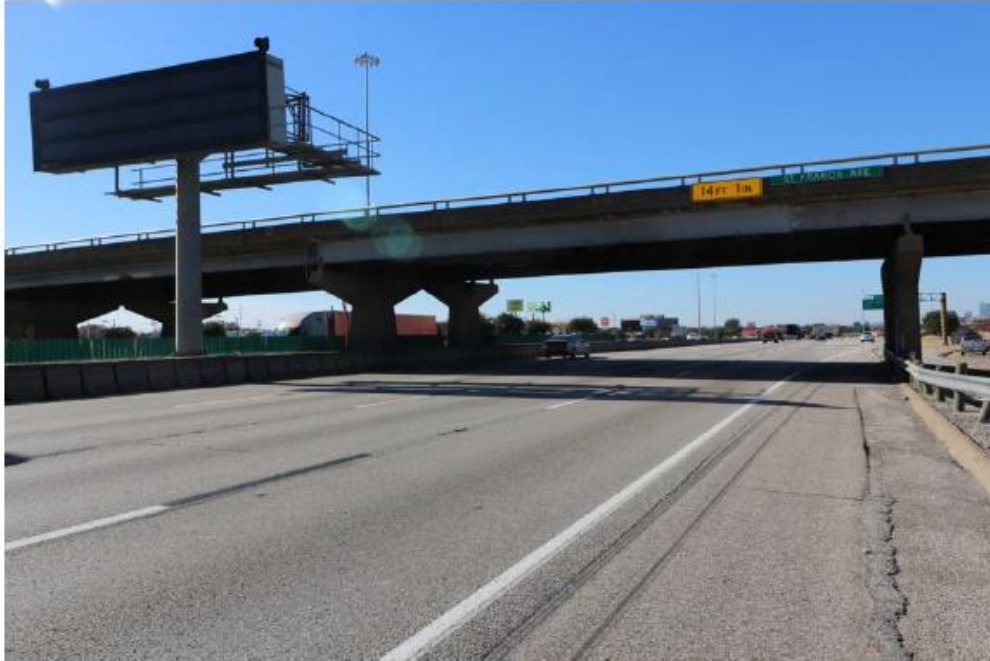
ROADWAY UNDER BRIDGE
