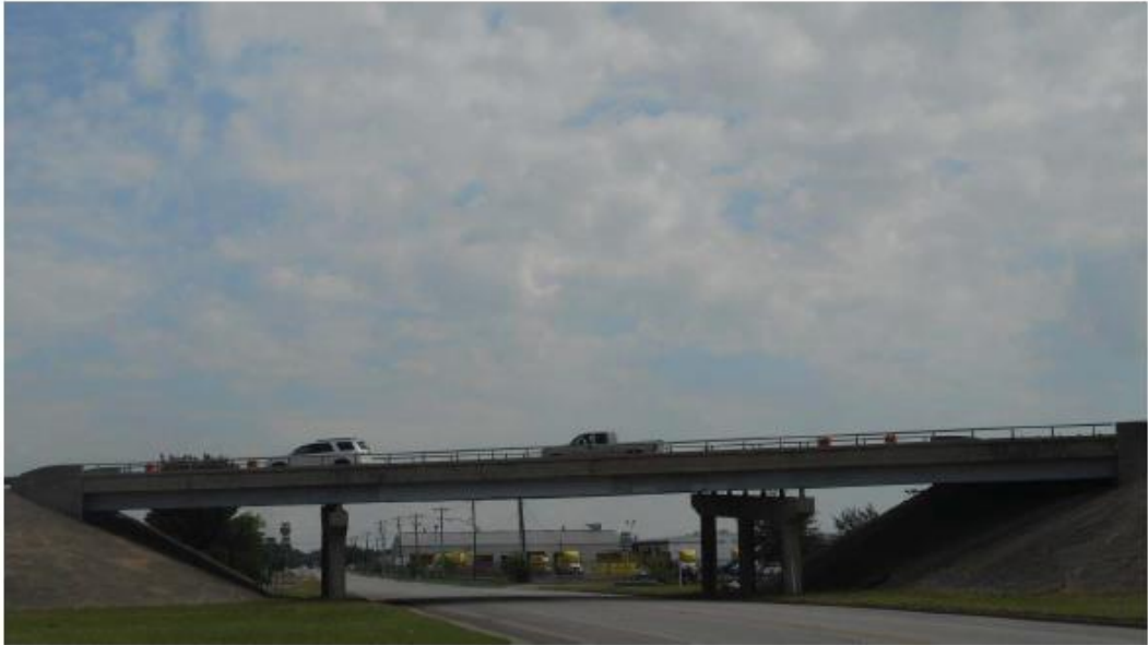
2 - Elevation looking East
