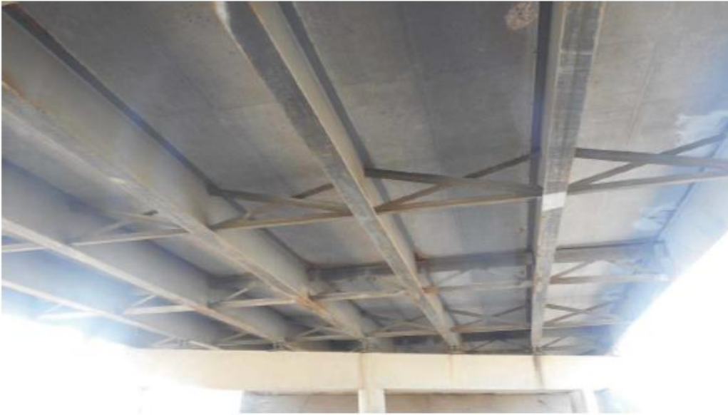
3 - Under looking South
