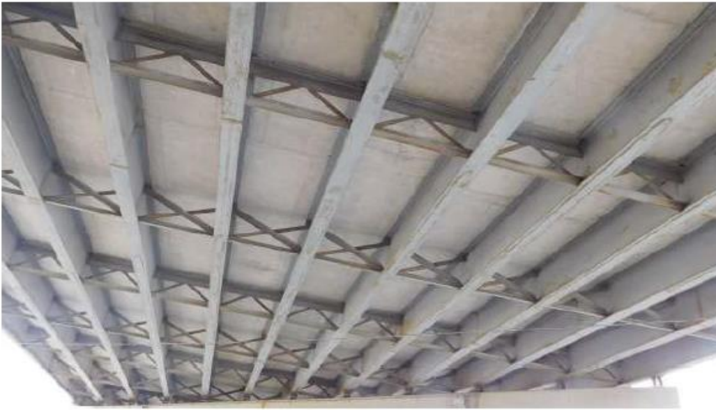
3 - Under looking South
