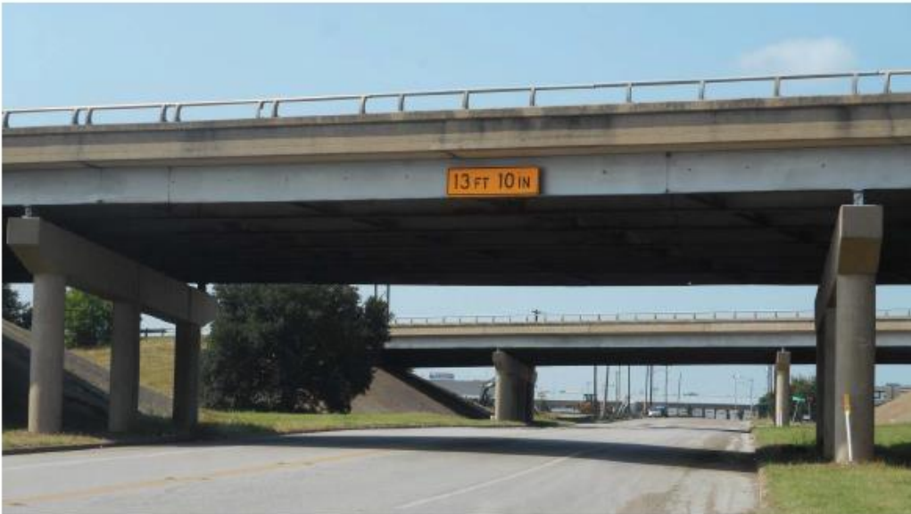
4 - Roadway Under looking West
