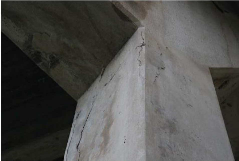
SOUTH COLUMN AT BENT 3
