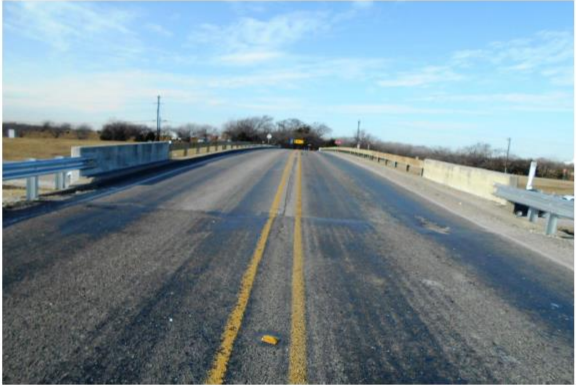
BRIDGE ROADWAY LOOKING WEST
