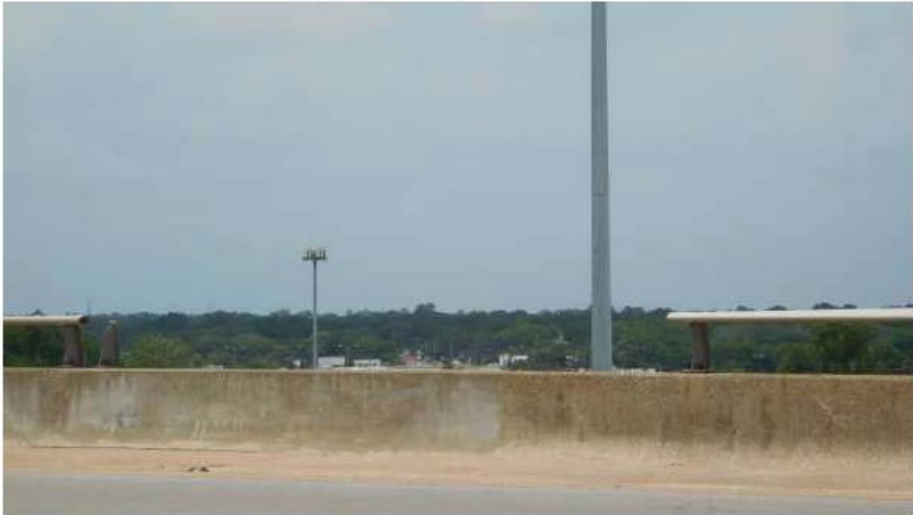
7 - Missing 20 ft tube section on East bridge rail
