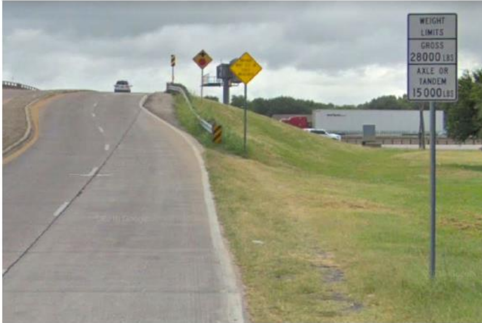
LOAD POSTING - SOUTH APPROACH
