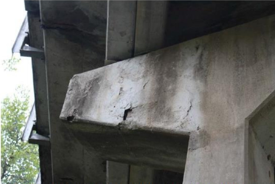
SOUTH END OF BENT CAP 2
