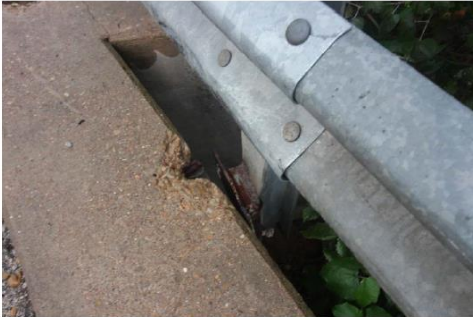
SOUTH CURB NEAR EAST BRIDGE END
