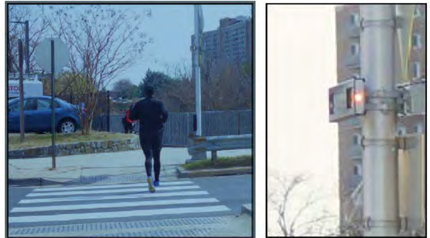
Figure 2. View of pilot light to pedestrian at shared-use path crossing with median refuge. Enlargement of pilot light at right.
