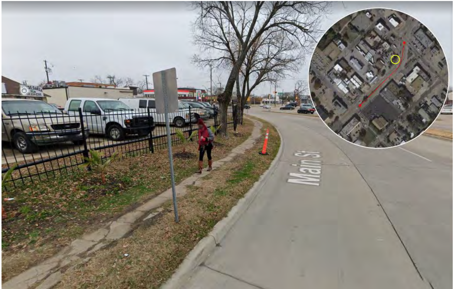
Figure 5: Pedestrian facilities approaching the intersection of Main St and Carroll lack ADA compliance. Sidewalk has been overrun by vegetation. Abutting property trees within the ROW.
