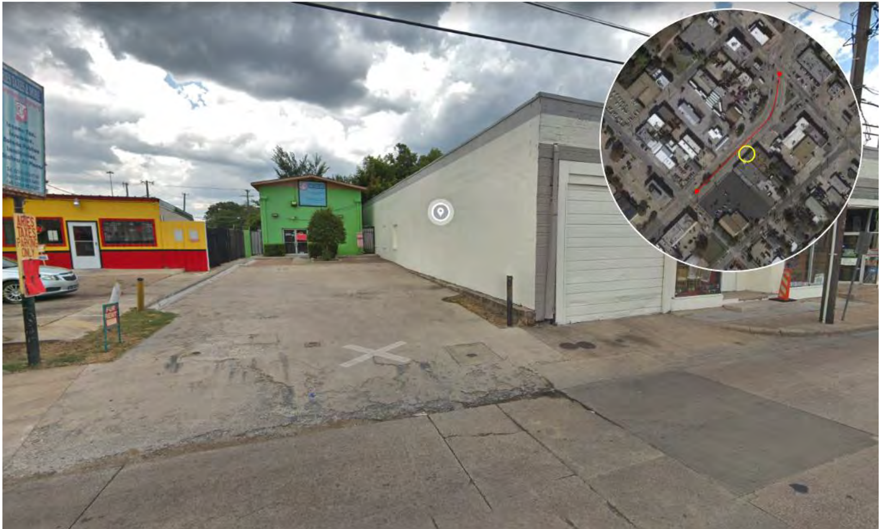
Figure 4: Access points and driveways with ADA compliance issues east side of Main St. Pedestrian facility is impeded upon by existing utilities and private driveways.
