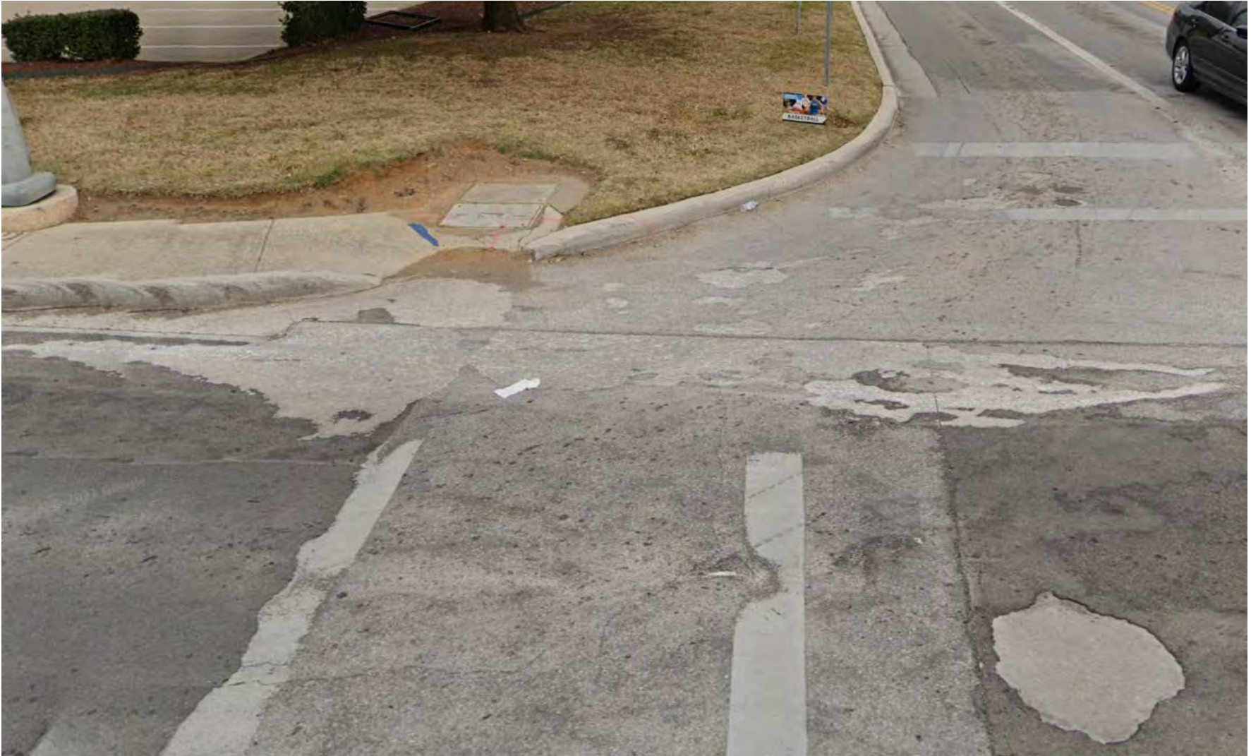
Figure 1: Pedestrian facilities at intersection of S Davis and Arkansas Ln: some sections lacking ADA compliance, no connected sidewalk facilities to Davis, utilities need to be relocated, narrow existing sidewalks, poor conditions, deficient crosswalk striping, etc.
