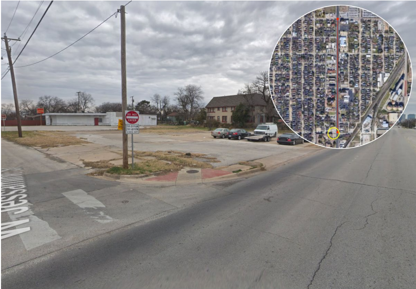
Figure 4: No connecting pedestrian facility on the corner of Jessamine and Hemphill, sidewalk is not ADA compliant. Vegetation has overrun much of the sidewalk. Road striping is deficient.
