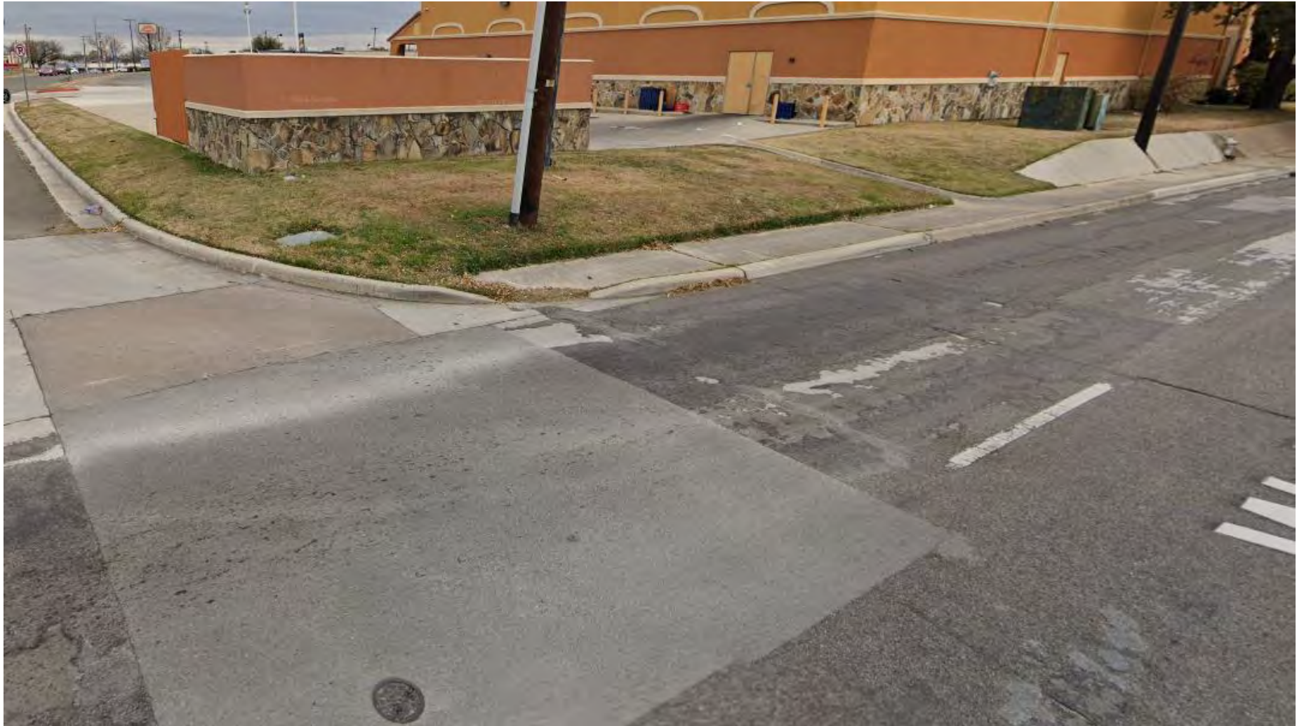
Figure 5: (Westbound along W Arkansas Ln) – More examples of access points with deficient conditions, lack of ADA compliance, limited right-of-way, and poor pavement conditions.
