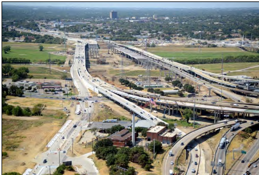
Figure 3-15: Reconstruction of I-30/I-35E Interchange
