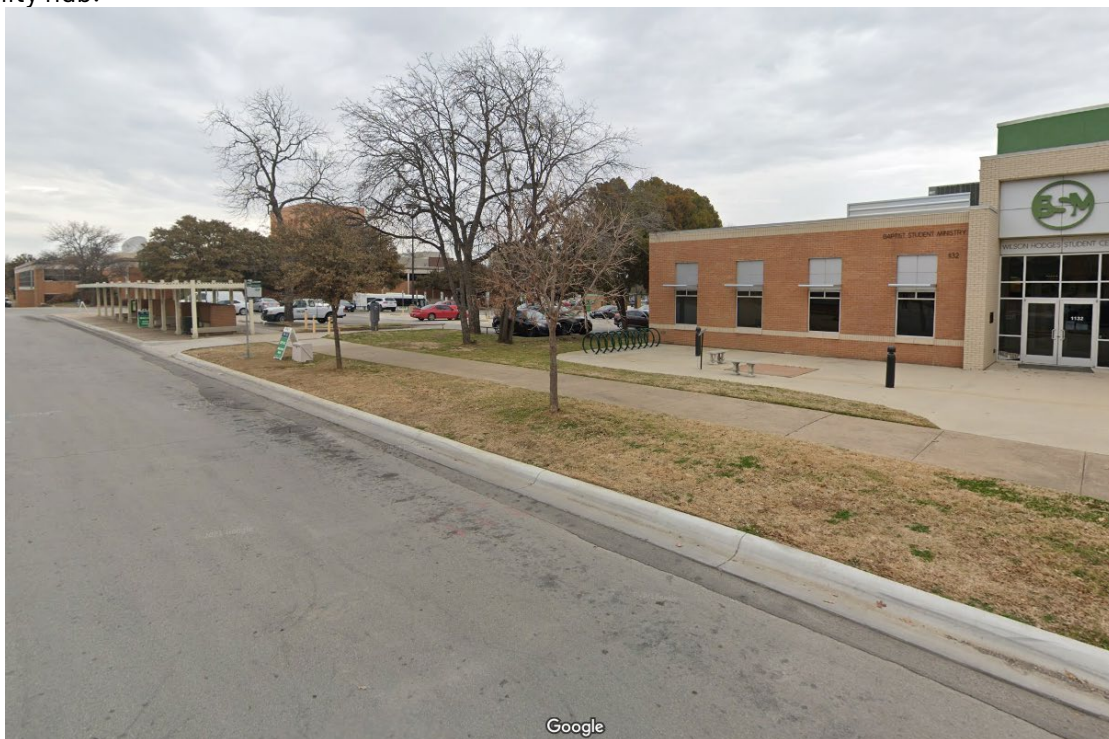
Figure 16: Union Transfer Center at UNT Denton (Google Maps)
