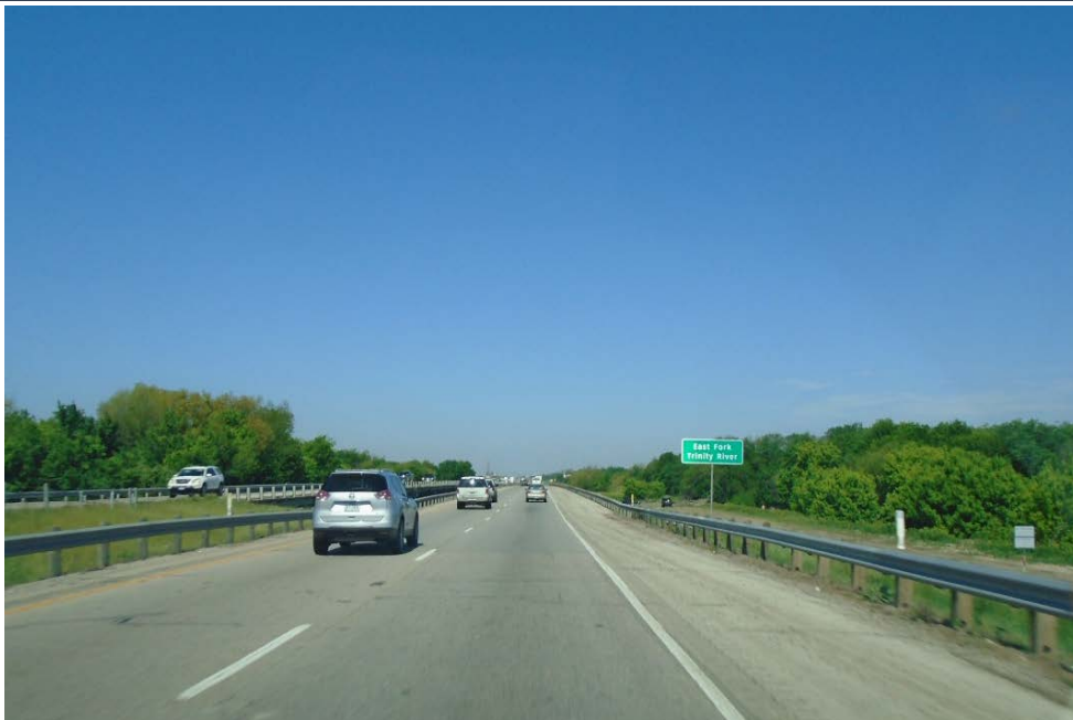
Photograph 22: View of existing westbound US 80 at the East Fork Trinity River. View is to the west. (4/26/2018)
