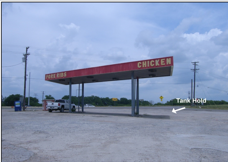
Photograph 16: View towards the tank hold of the former County Line Truck Stop (Currently Shorty's Texas Bar B Q) LPST, PST site at 780 E. US 80, Sunnyvale. View is to the east-northeast. (6/12/18)
