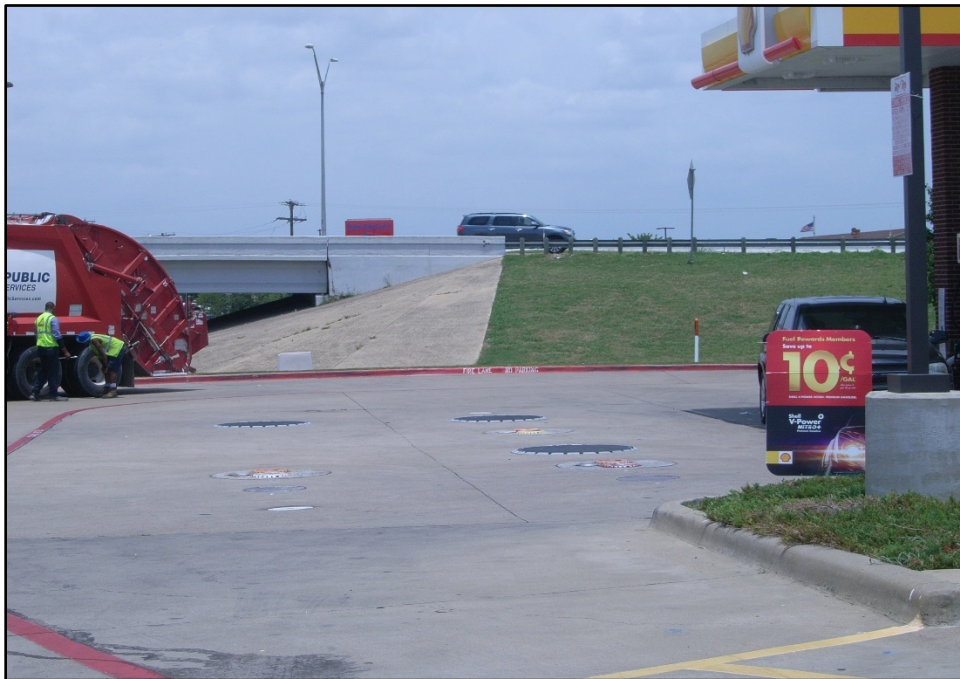
Photograph 15: View towards the tank hold of the Shell 100970 LPST, PST site at 106 E. US 80, Mesquite, TX. The eastbound US 80 frontage road is in the background of the photo. ROW would be acquired from this site. View is to the north. (6/12/18)
