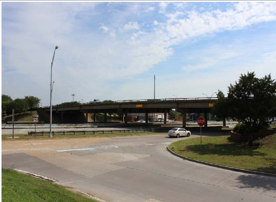
Photograph 2: View of Big Town Boulevard Bridge. View is to the northeast. (8/28/17)
