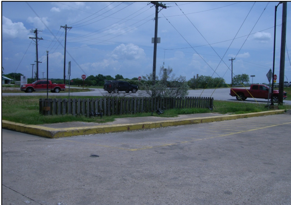
Photograph 23: View towards one of two tank holds at the Knox Super Stop PST site at 14410 US 80, Forney, TX. This tank hold is located near the southeast corner of the site. No ROW would be acquired from this site. View is to the south-southeast (6/12/18)
