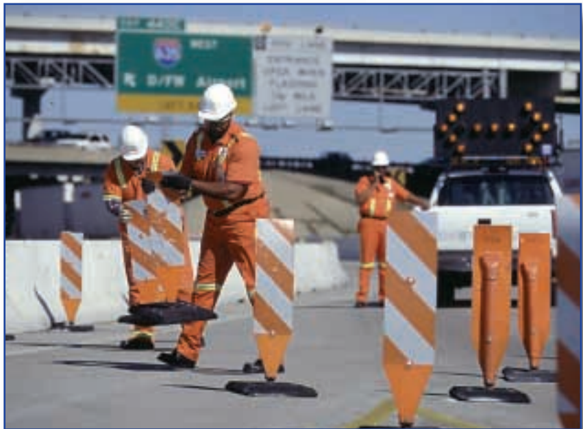
Operation of the Interstate Highway 35E (Stemmons Freeway) immediate-action HOV facility involves the opening and closing of access ramps.
