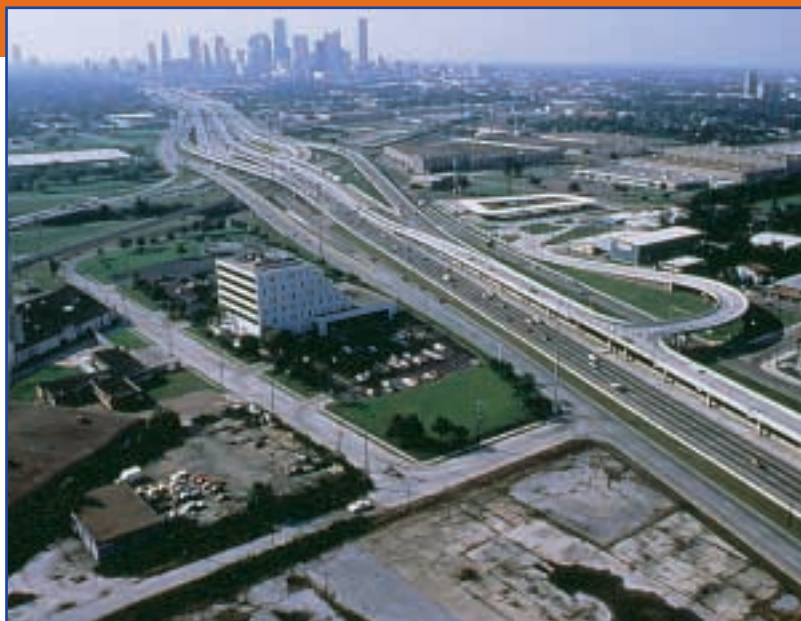
Barrier-separated HOV lanes with flyover ramps along Houston's Interstate Highway 45 (Gulf Freeway). Flyover ramps are an alternative form of egress/ingress access to HOV facilities.
