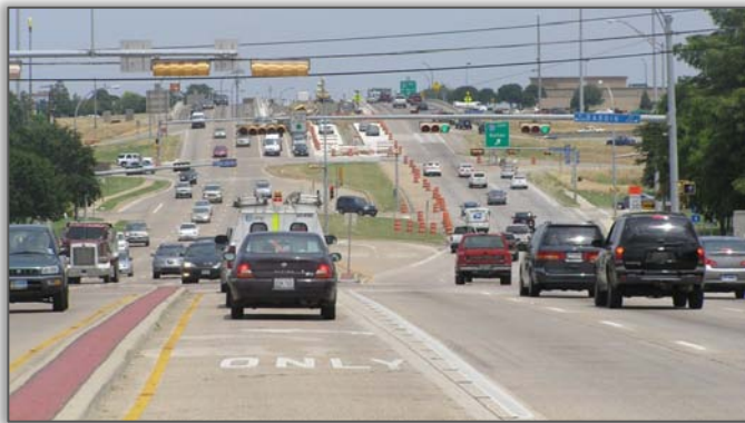
Intersection Improvement at Cooper Street and IH 20, Arlington, TX
