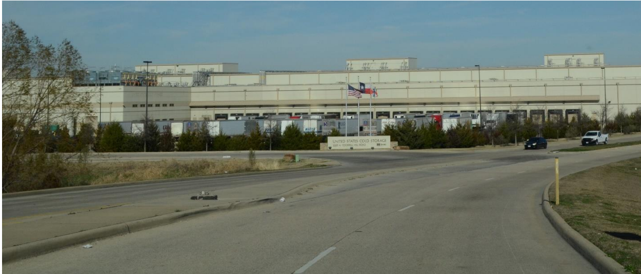
Image 1: Warehousing in North Central Texas
