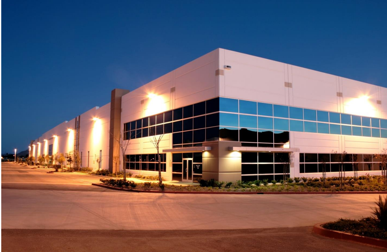
Image 2: Warehouse with Improved Façade
