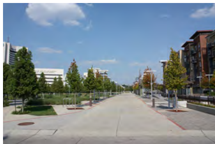
Figure 5.23: Open space around transit station, Baylor UMC Station (Photo by T. R. Ozdil, 2010)
