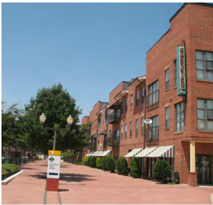
Figure 3.14: Image of new multifamily residential in Downtown Plano (Source: T. R. Ozdil, 2009)
