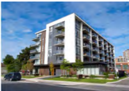
Figure 2.36: Port street condominiums (Source: City of Toronto, 2010)
