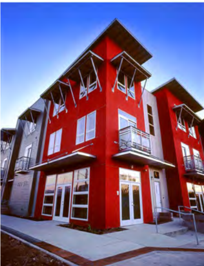
Figure 2.46: Building in Salttilo Lofts (Source: Architecture365, 2009)
