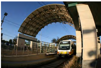
Figure 3.44: Downtown rail station (Source: 5th Street Crossing, 2008)
