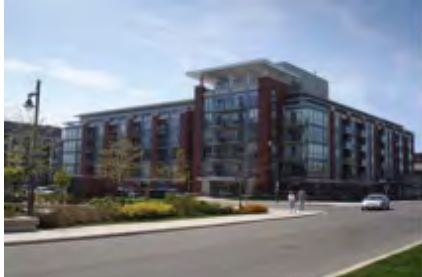
Figure 2.35: Port street condominiums (Source: City of Toronto, 2010)
