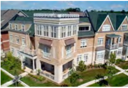
Figure 2.33: Townhouses (Source: City of Toronto, 2010)
