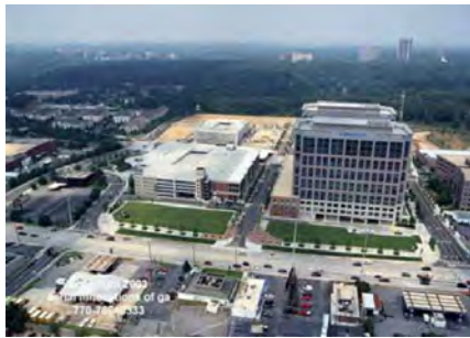
Figure 2.22: The construction of Lindbergh city center (Source: Lindbergh City, 2009)
