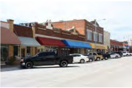
Figure 3.33: Image of downtown Garland (Source D.S. Cooper, 2009)
