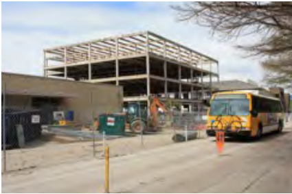
Figure 3.42: Parking garage (Source: D.S. Cooper, 2009)
