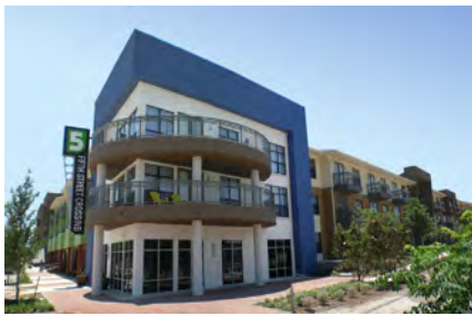
Figure 3.43: Photo of 5th Street Crossing (Source: D.S. Cooper)
