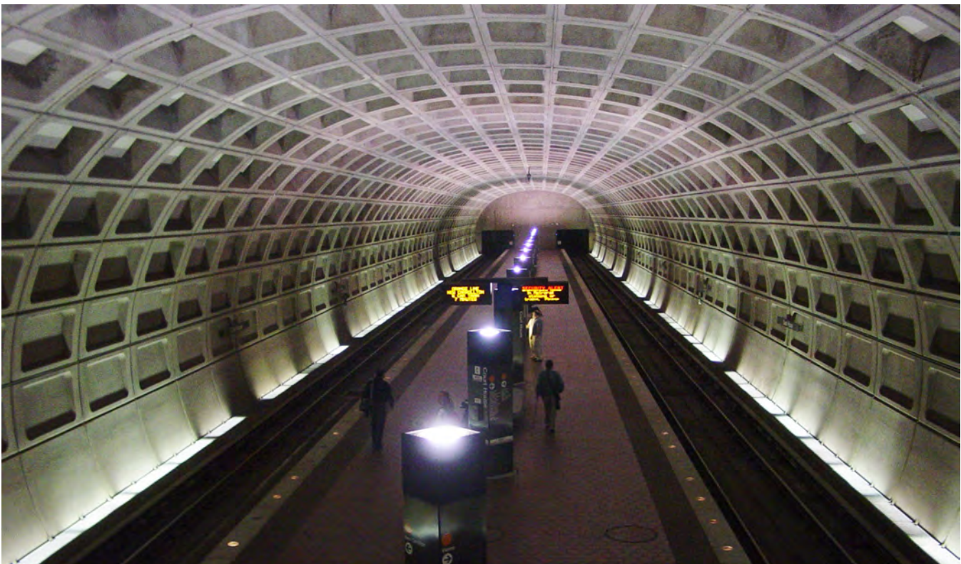
Figure 3.5: Image of Court House Metro Station (Source: Wikipedia, 2010)
