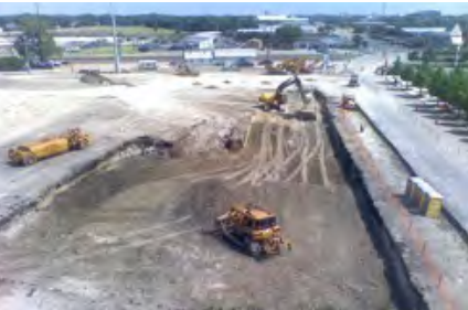
Figure 3.35: Site construction (Source: City of Garland, 2009)
