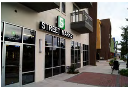
Figure 3.49: 5th Street Market (Source: Brown, 2010)
