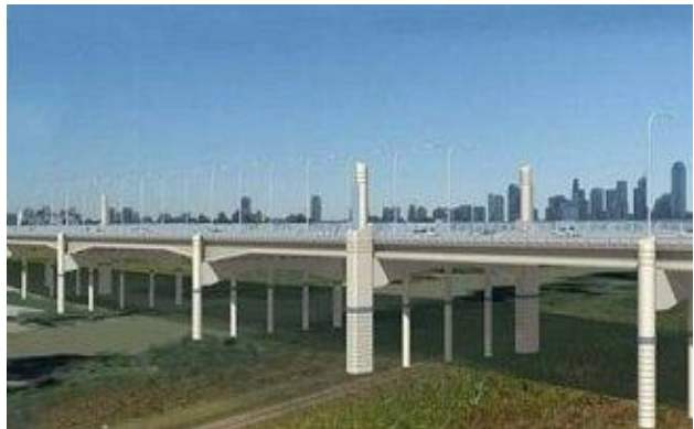
Figure 18: New Sylvan Avenue Bridge
