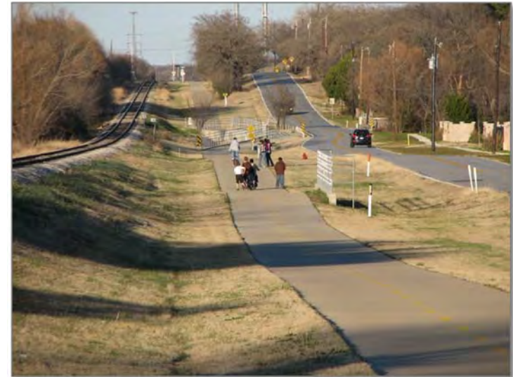
FIGURE 24: SHARED-USE PATH, NORTH RICHLAND HILLS, TX
