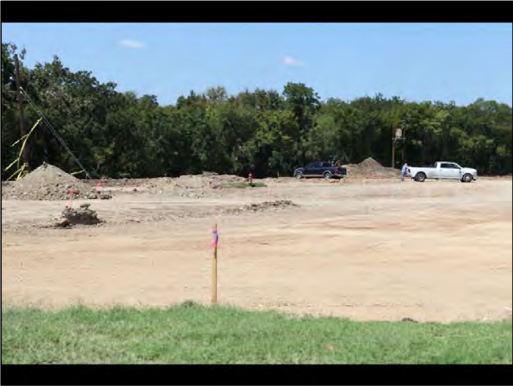
199 and 183 intersection: new Quick Trip gas station.
