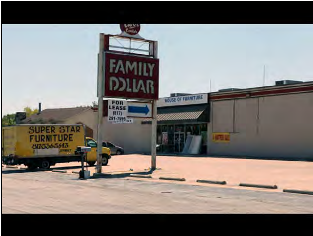
Tour of Highway 199 corridor: typical building along 199 corridor. The ambiguous street edge does not encourage safe traffic flow and lacks pedestrian and bicycle facilities. The large signage is oriented to automobile traffic and is not a human scale.
