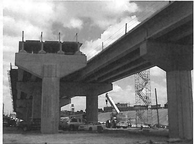
Construction on the I-30/SH 360 Interchange Project in Arlington. The $233 million project will increase safety, connectivity and mobility for motorists.
