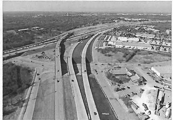
SH 121/360 interchange construction
