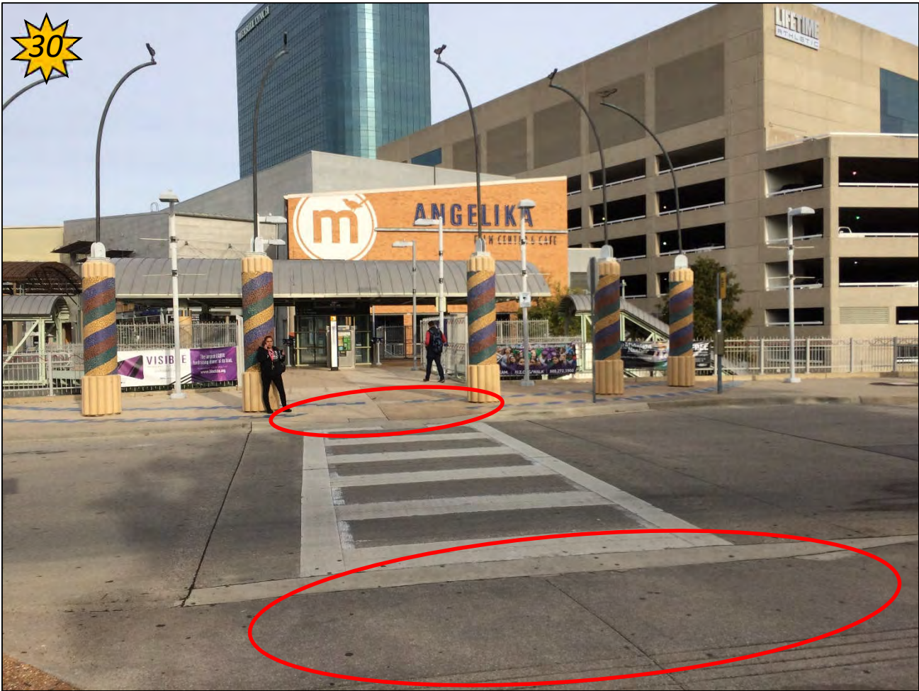
Add detectable warning surfaces to pedestrian ramps where missing. The above location is one example. Several others exist throughout the station area.
