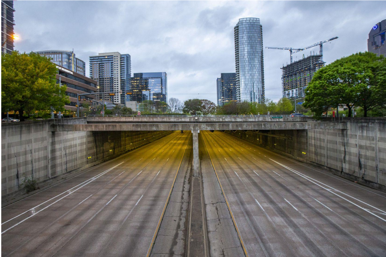
Figure 5. Woodall Rogers Freeway at 7:26 AM Tuesday, March 24, 2020
