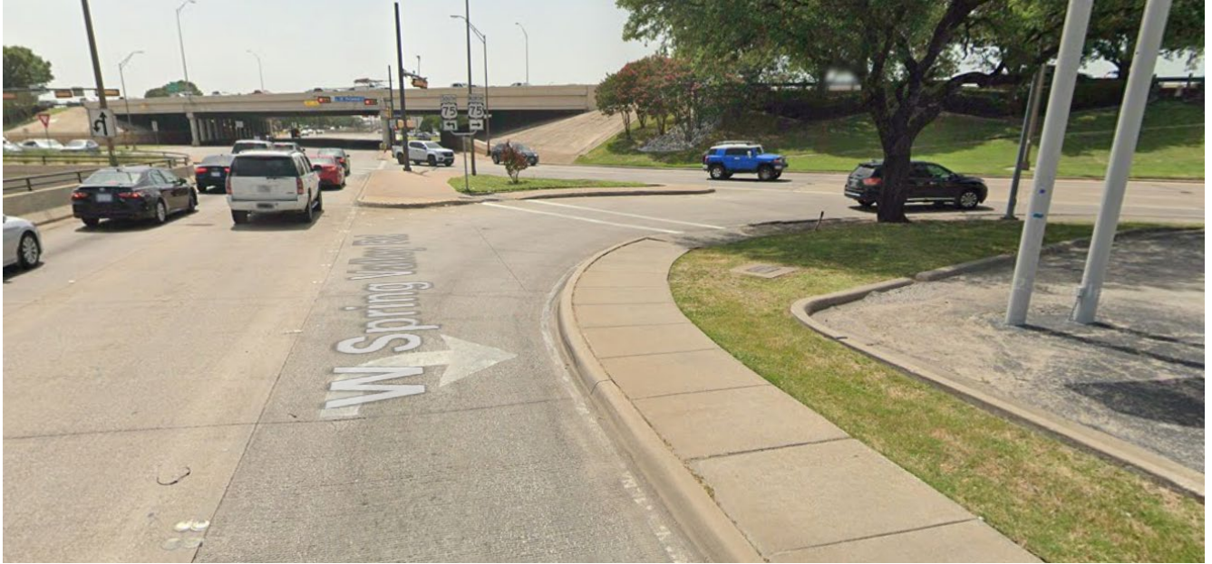
Figure 25: Design of northeast corner allows for high speed turns with reduced yielding to pedestrians
