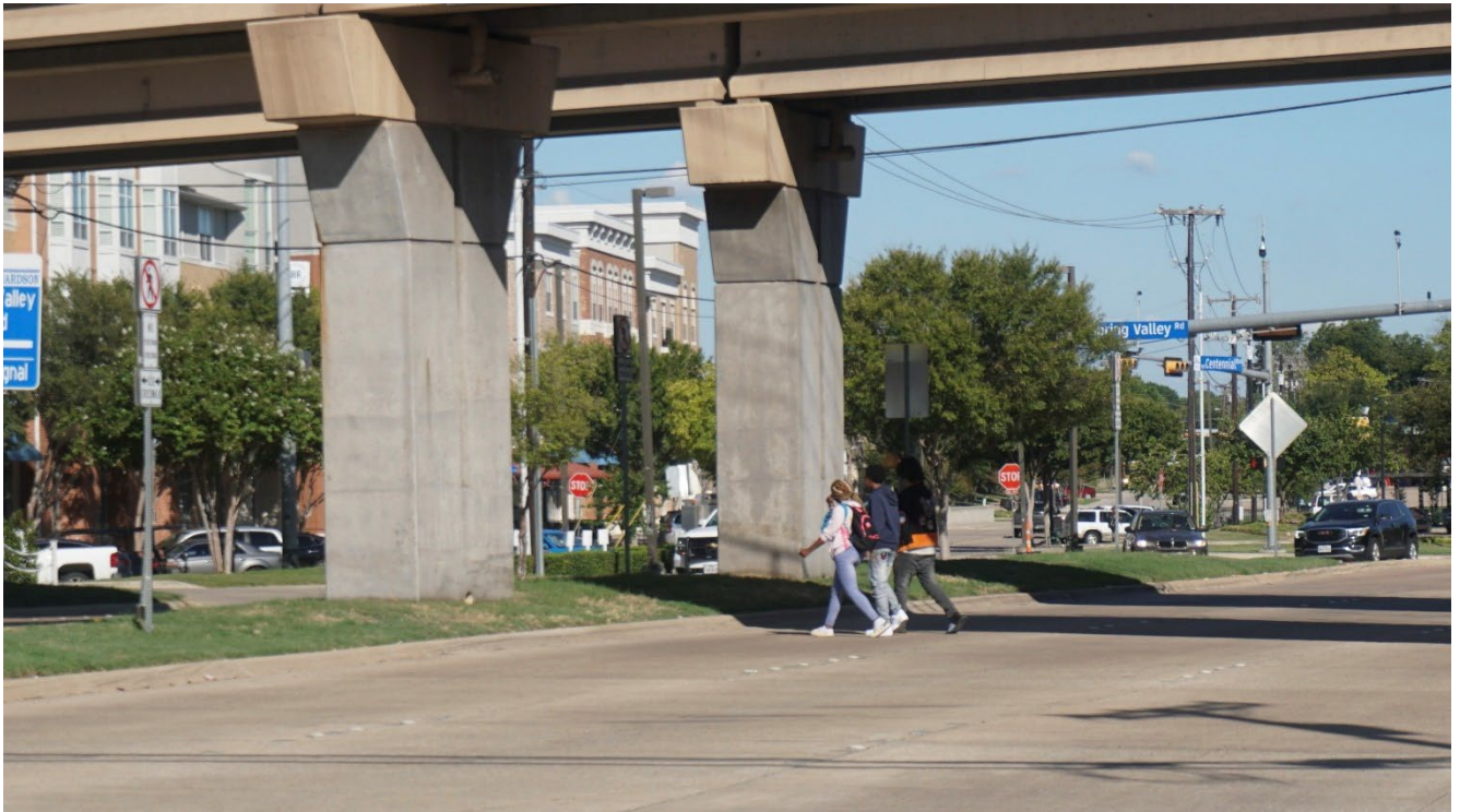
Figure 29: Some marked crosswalks were not within natural or expected paths
