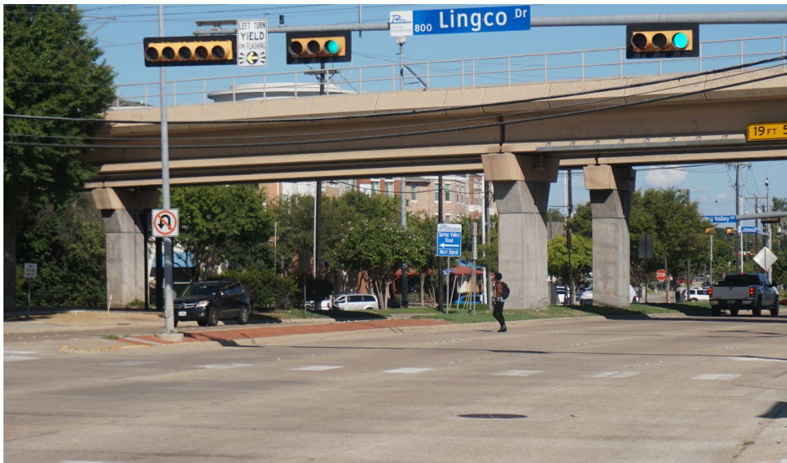
Figure 5: Some marked crosswalks were not within natural or expected paths
