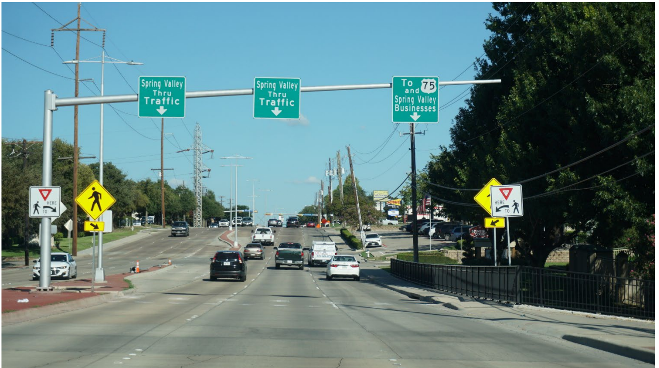
Figure 21: Eastbound overhead sign structure
