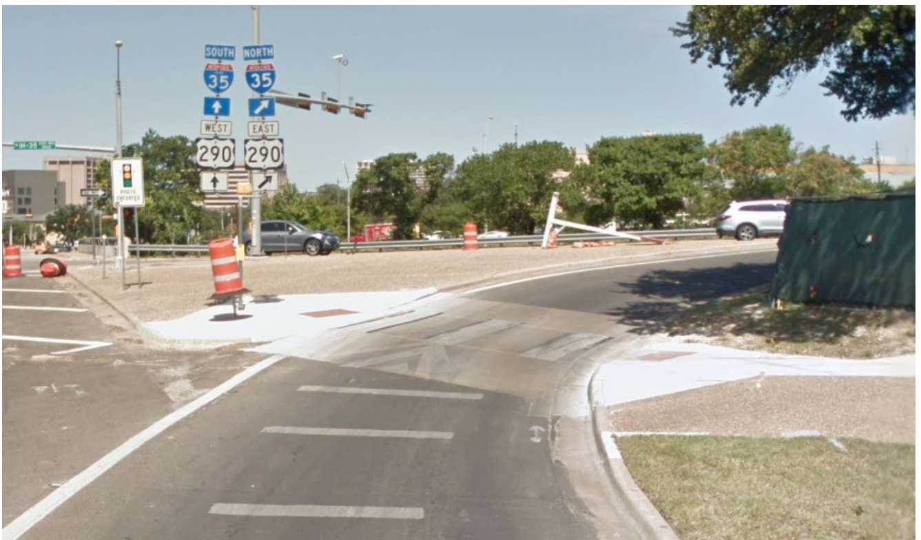
Figure 26: Example of a raised crosswalk on a turn lane joining an Interstate frontage road in Austin, TX ( Google StreetView )
