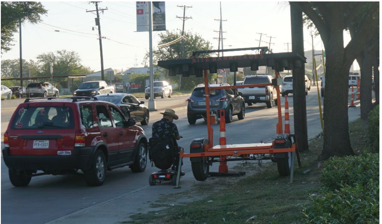
Figure 10: Closure of sidewalk with no warning or accessible detour path, located immediately adjacent to bus shelter
