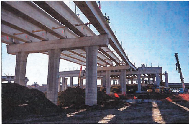
Above: Precast beams for direct connector bridge at SH 183
