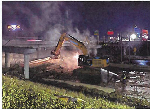
At Left: Bridge demolition
